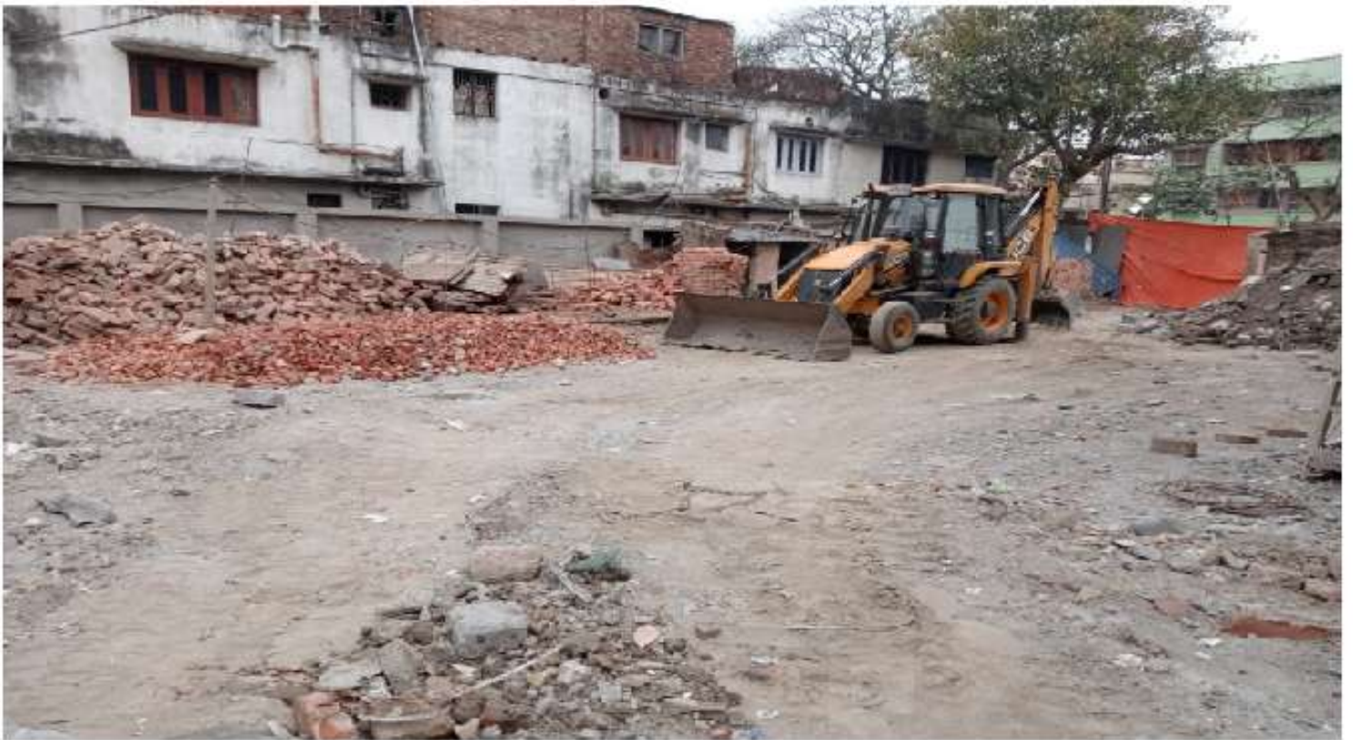
DRIVEWAY CONSTRUCTION IN PROGRESS
