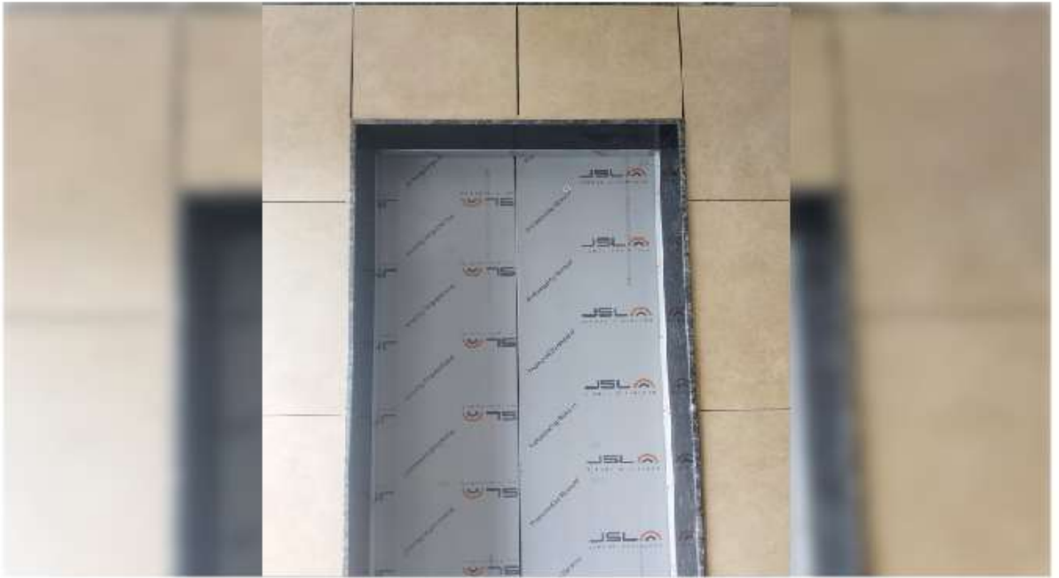
LIFT INSTALLATION IN PROGRESS
