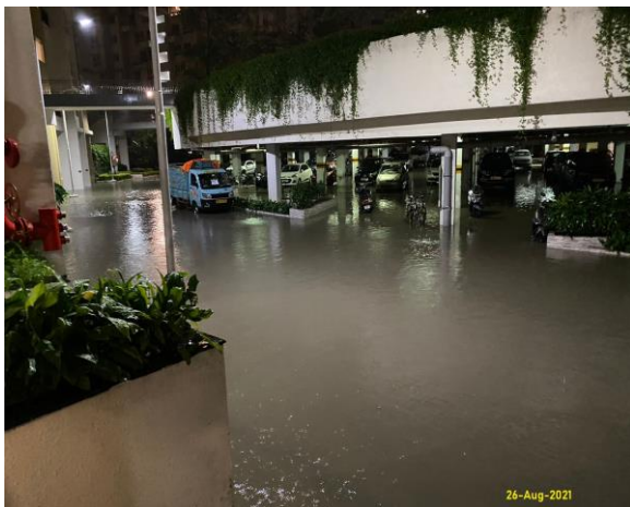
Faulty Drainage System leads to water log
