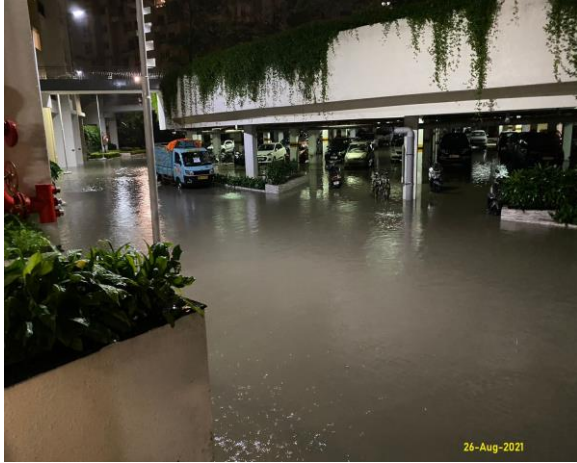
Faulty Drainage System leads to water log
