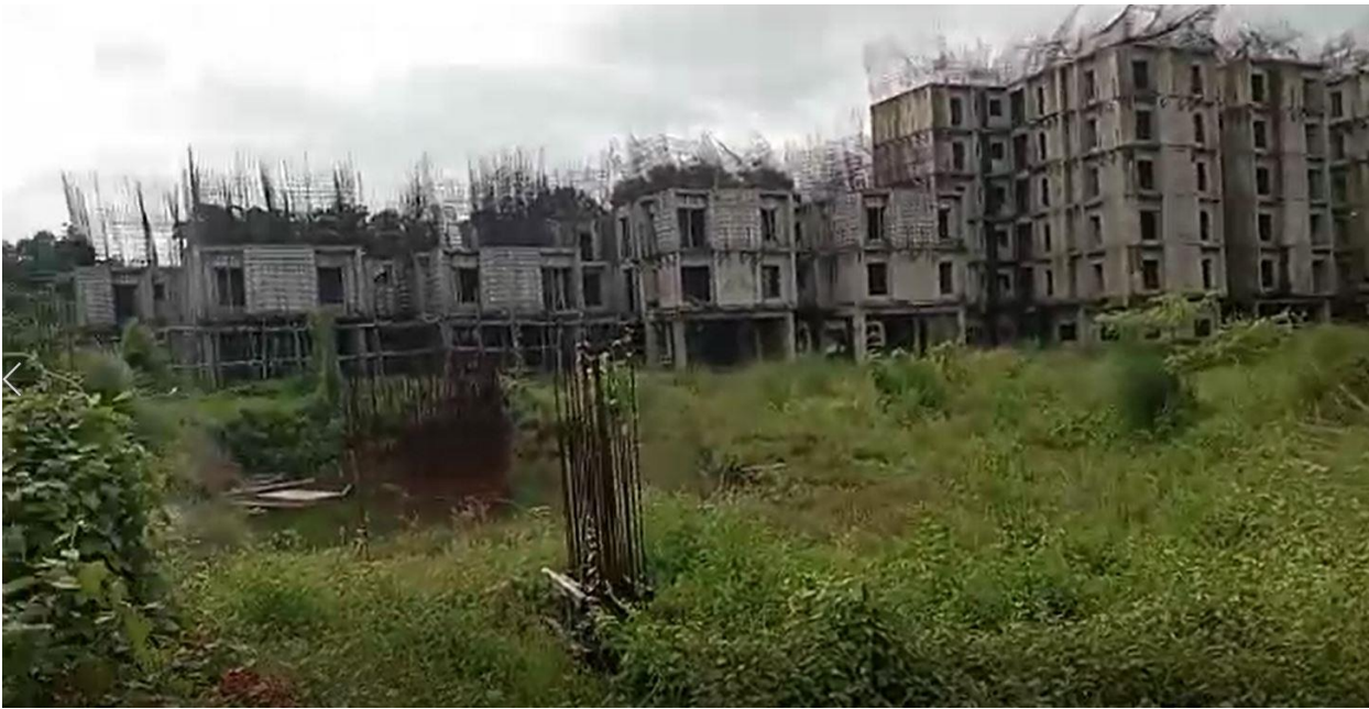
Water logging in foundations
