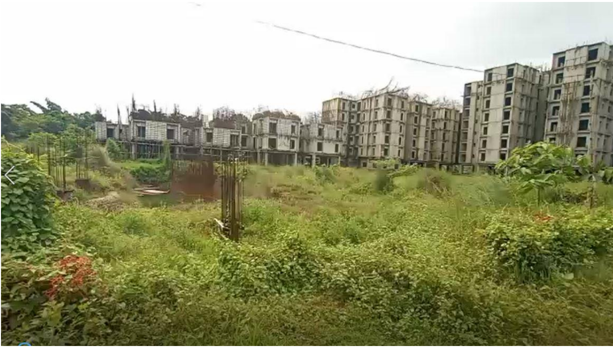
Ponds & water logging in foundations for last 1 year
