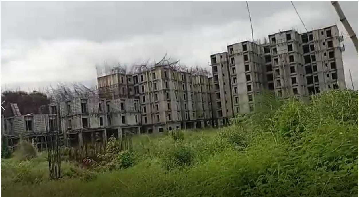
Ponds inside incomplete foundation Base
