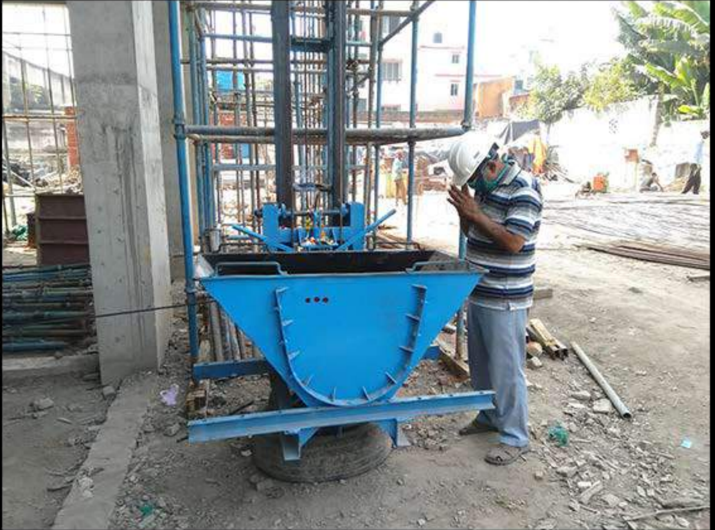
Material Hoist Install in the Site
