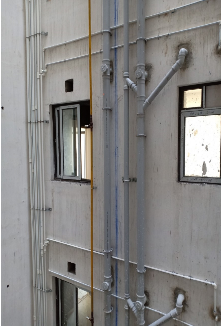
INTERNAL STORM & SEWER LINE
