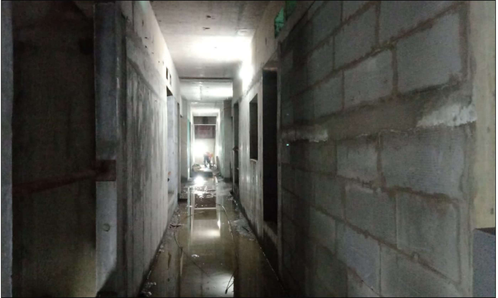
1 st Floor works under progress
