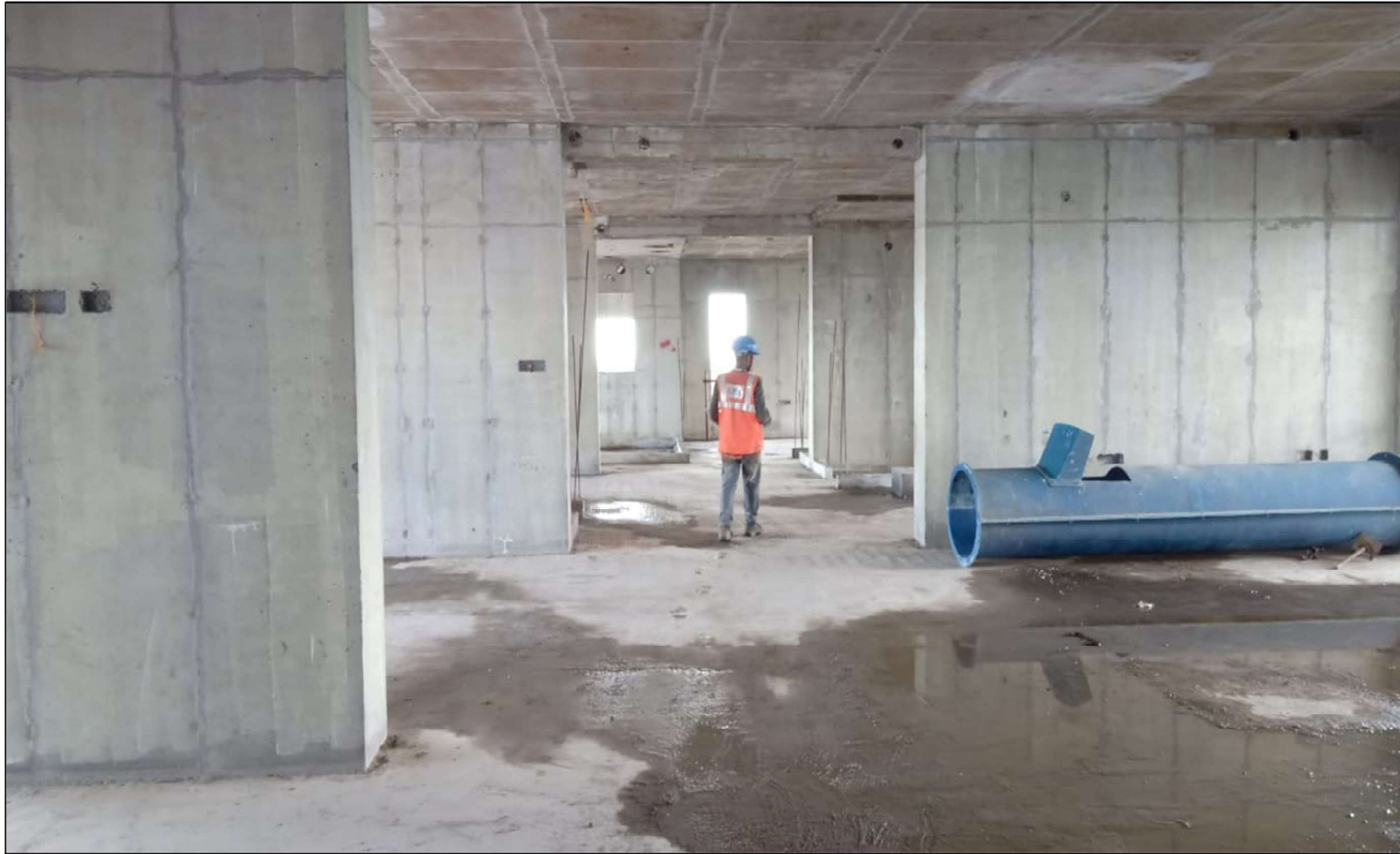
10 th Floor works under progress
