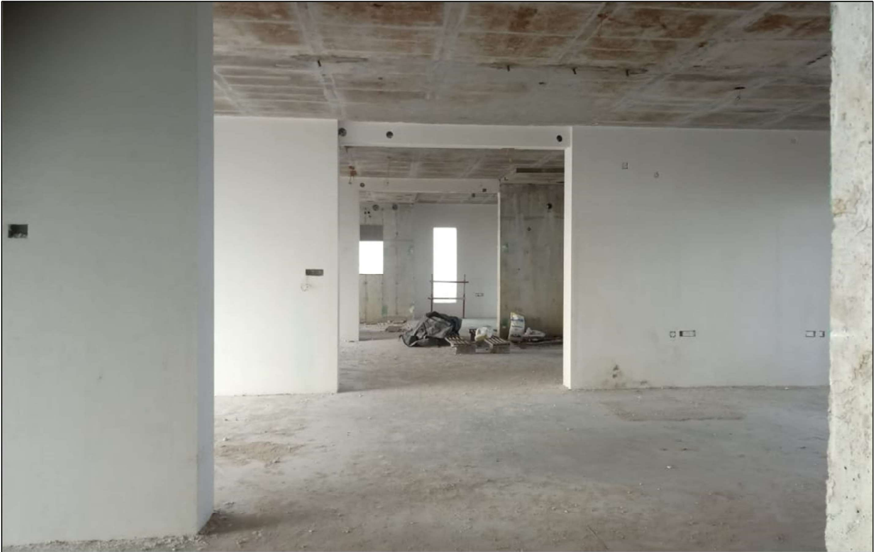
11 th Floor works under progress
