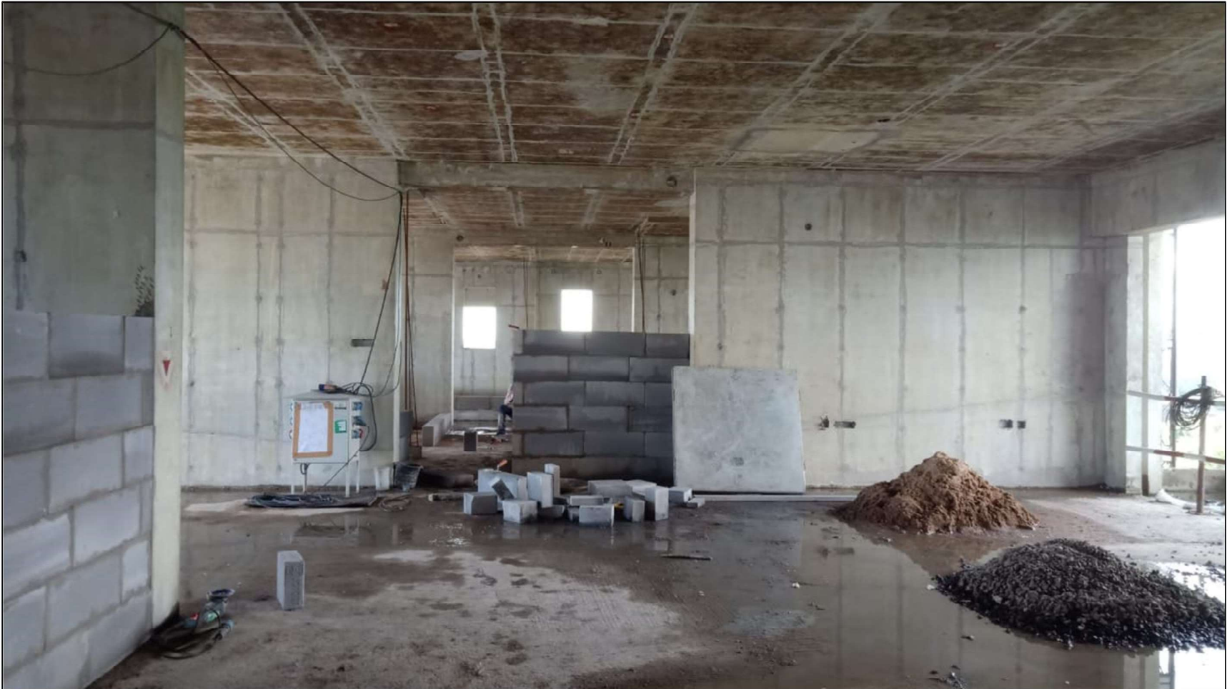
12 th Floor works under progress
