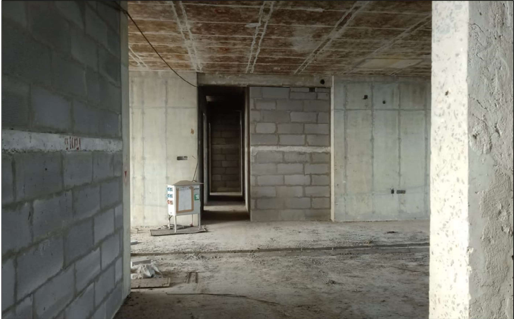
12 th Floor works under progress
