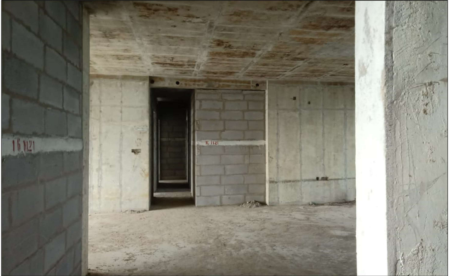
13 th Floor works under progress
