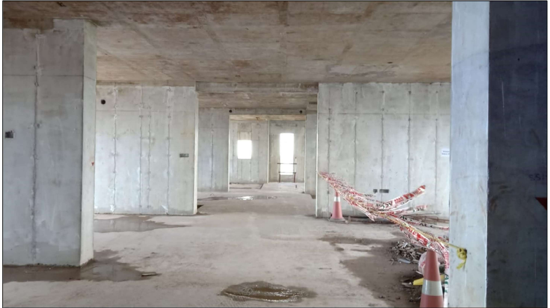
14 th Floor works under progress
