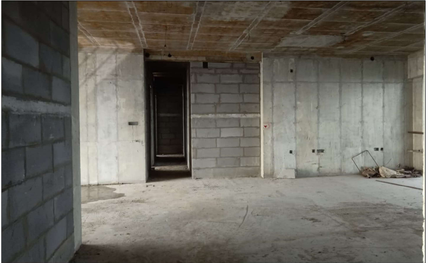
14 th Floor works under progress
