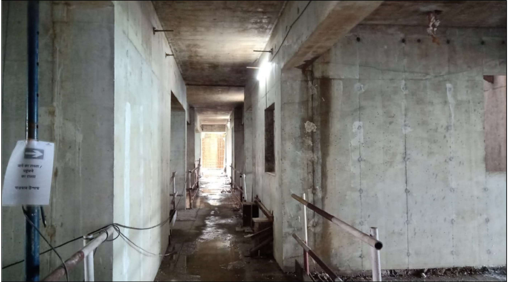
15 th Floor works under progress
