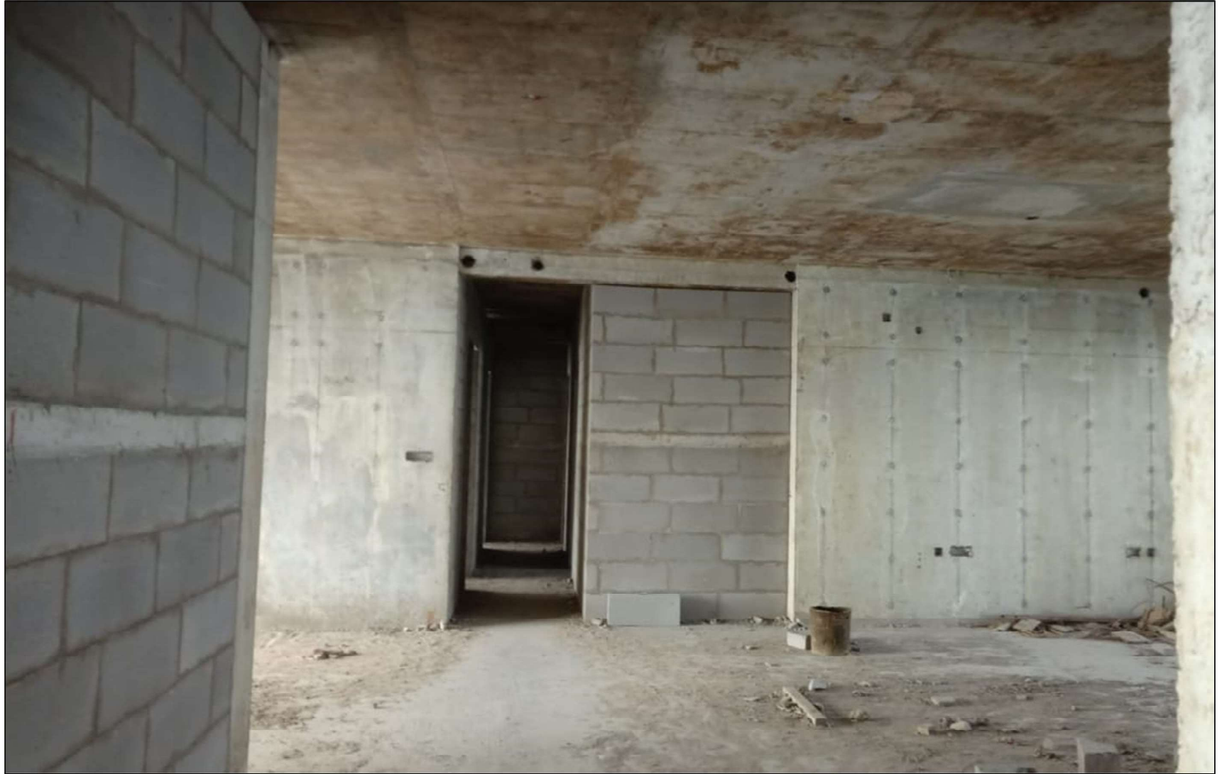
17 th Floor works under progress
