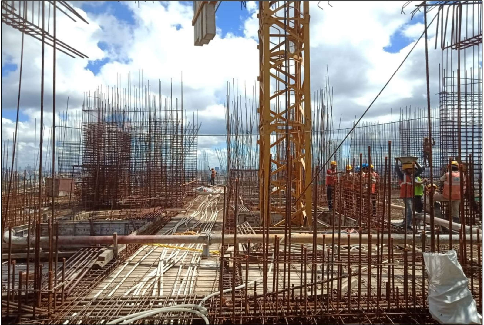
18 th Floor works under progress
