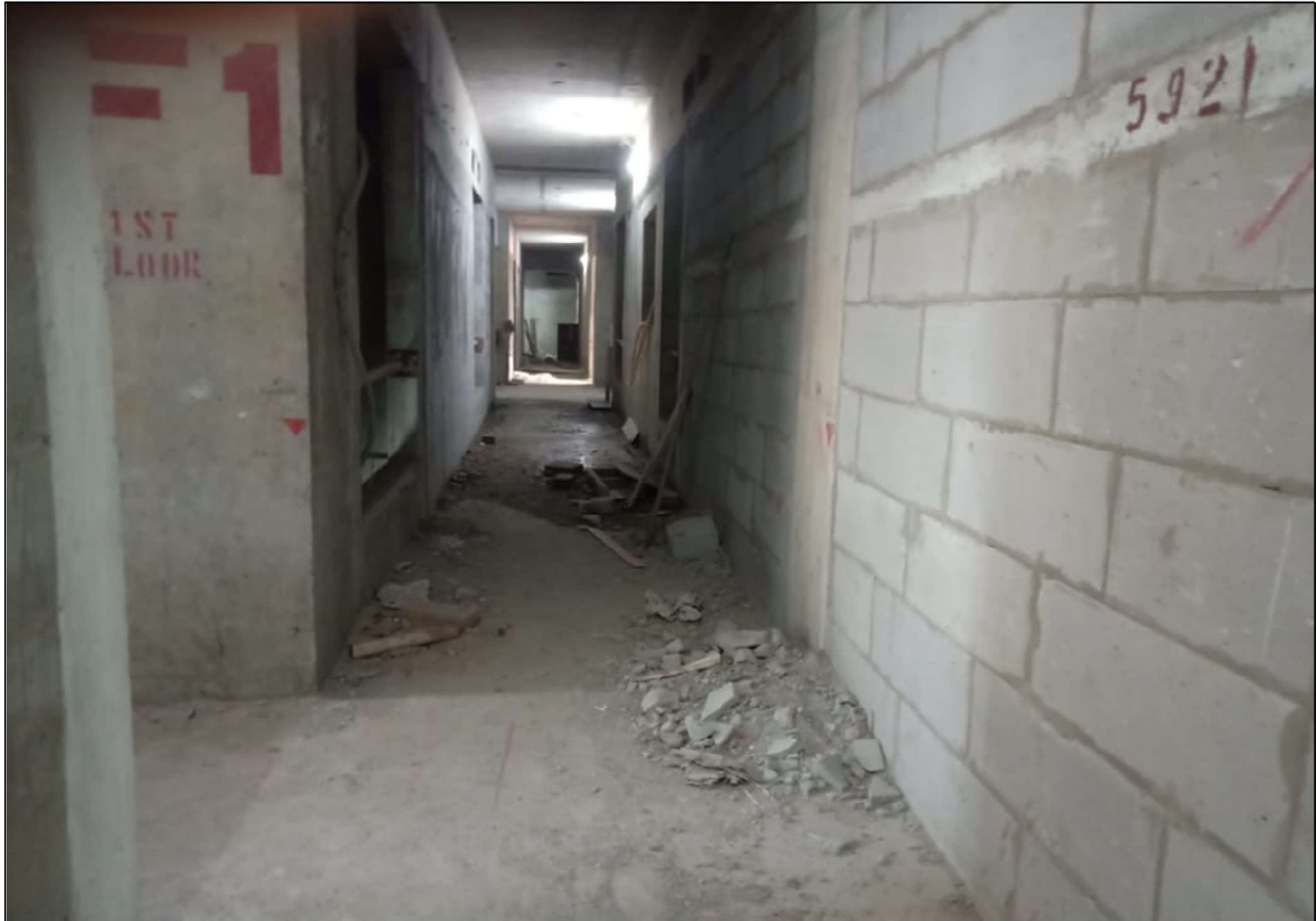
1 st Floor works under progress
