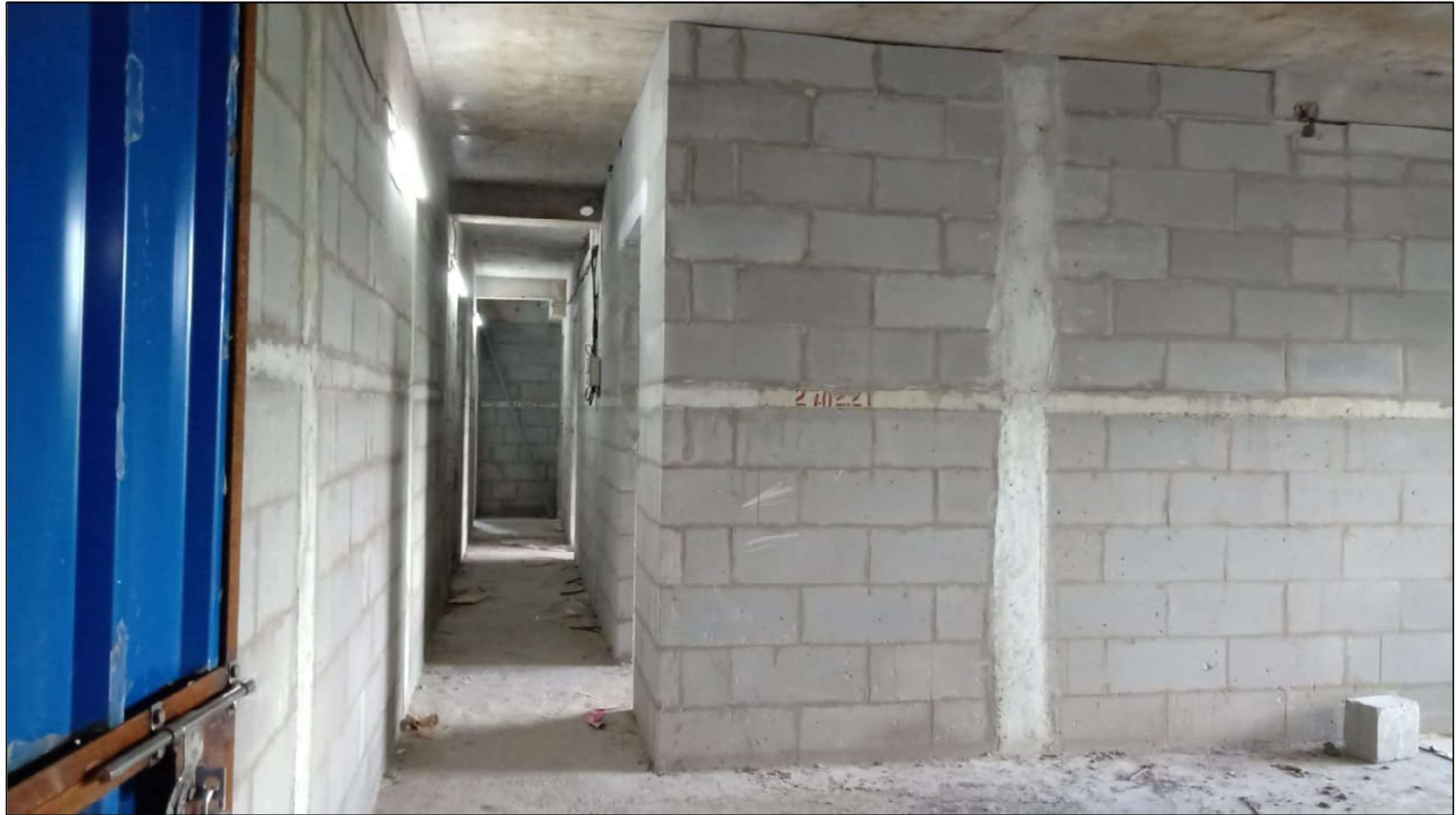
2 nd Floor works under progress
