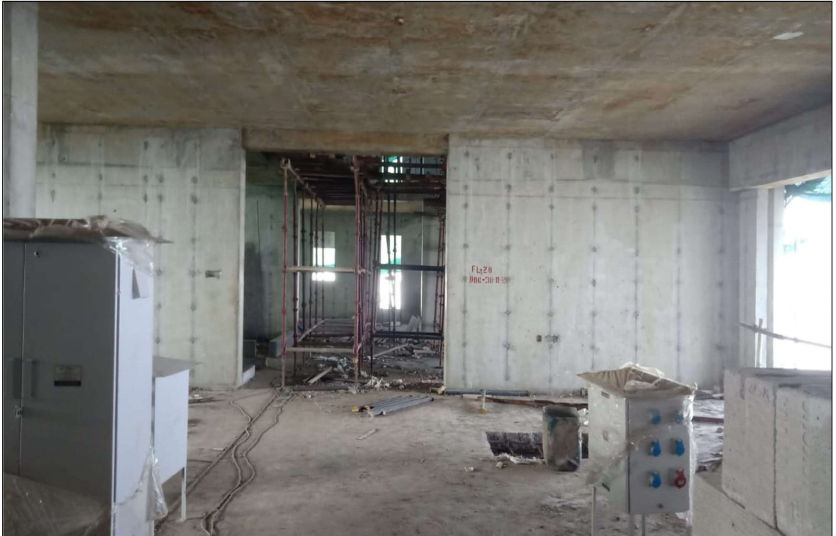
20 th Floor works under progress
