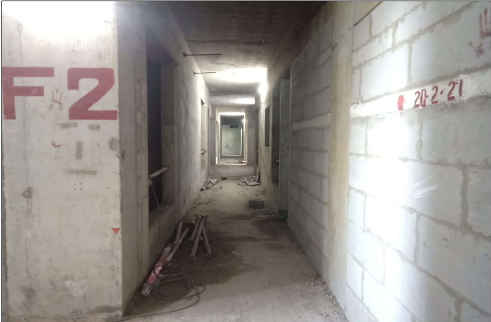
2 nd Floor works under progress
