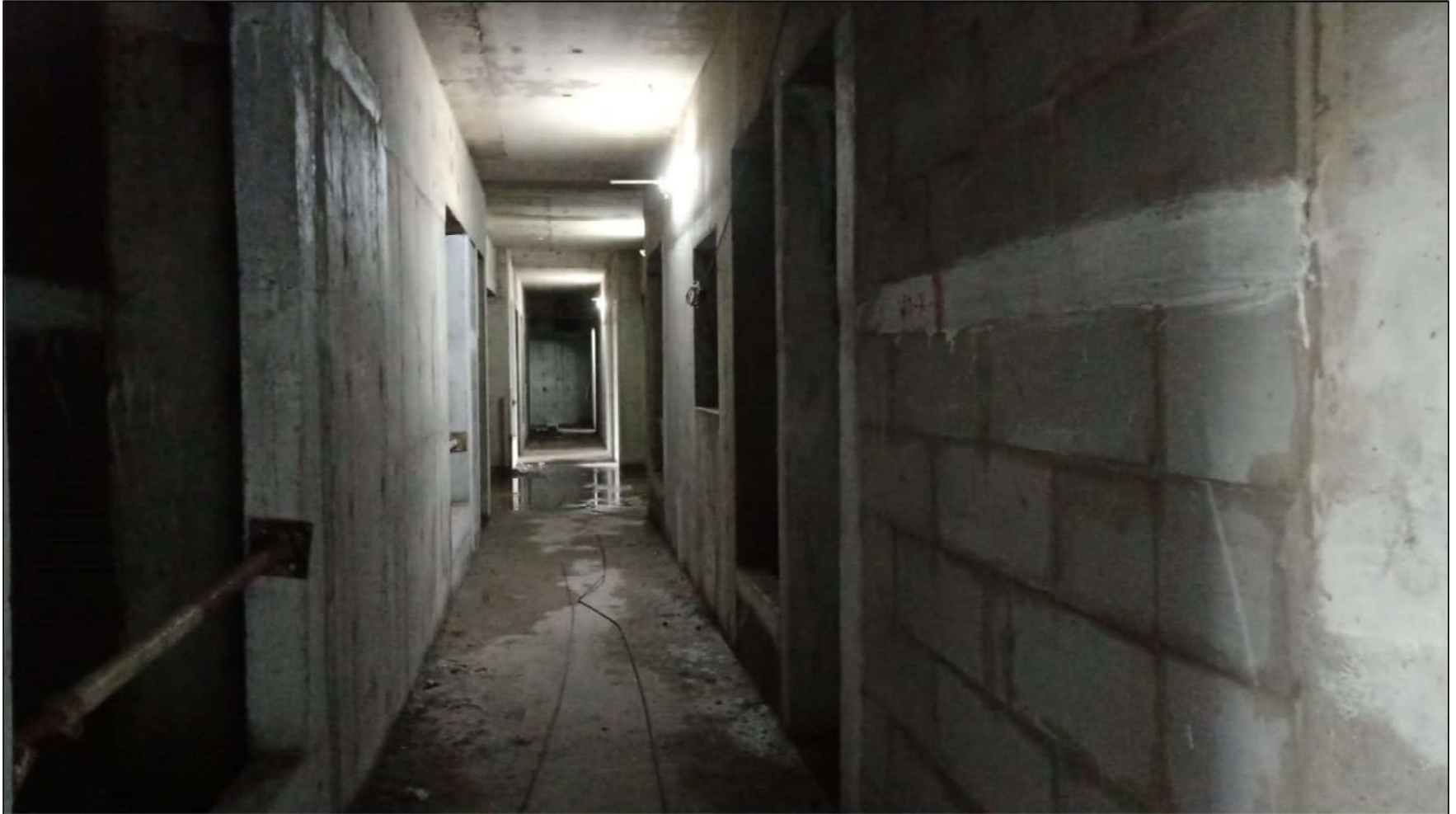
3 rd Floor works under progress
