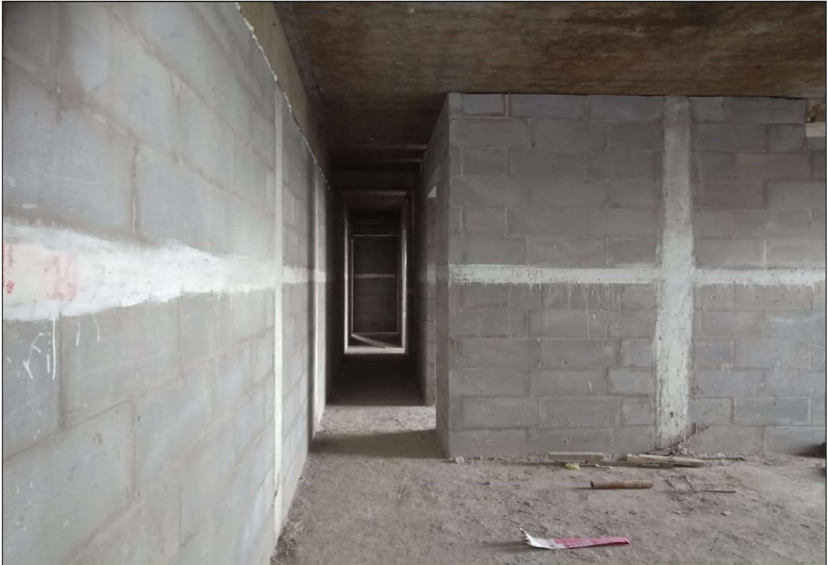
4 th Floor works under progress
