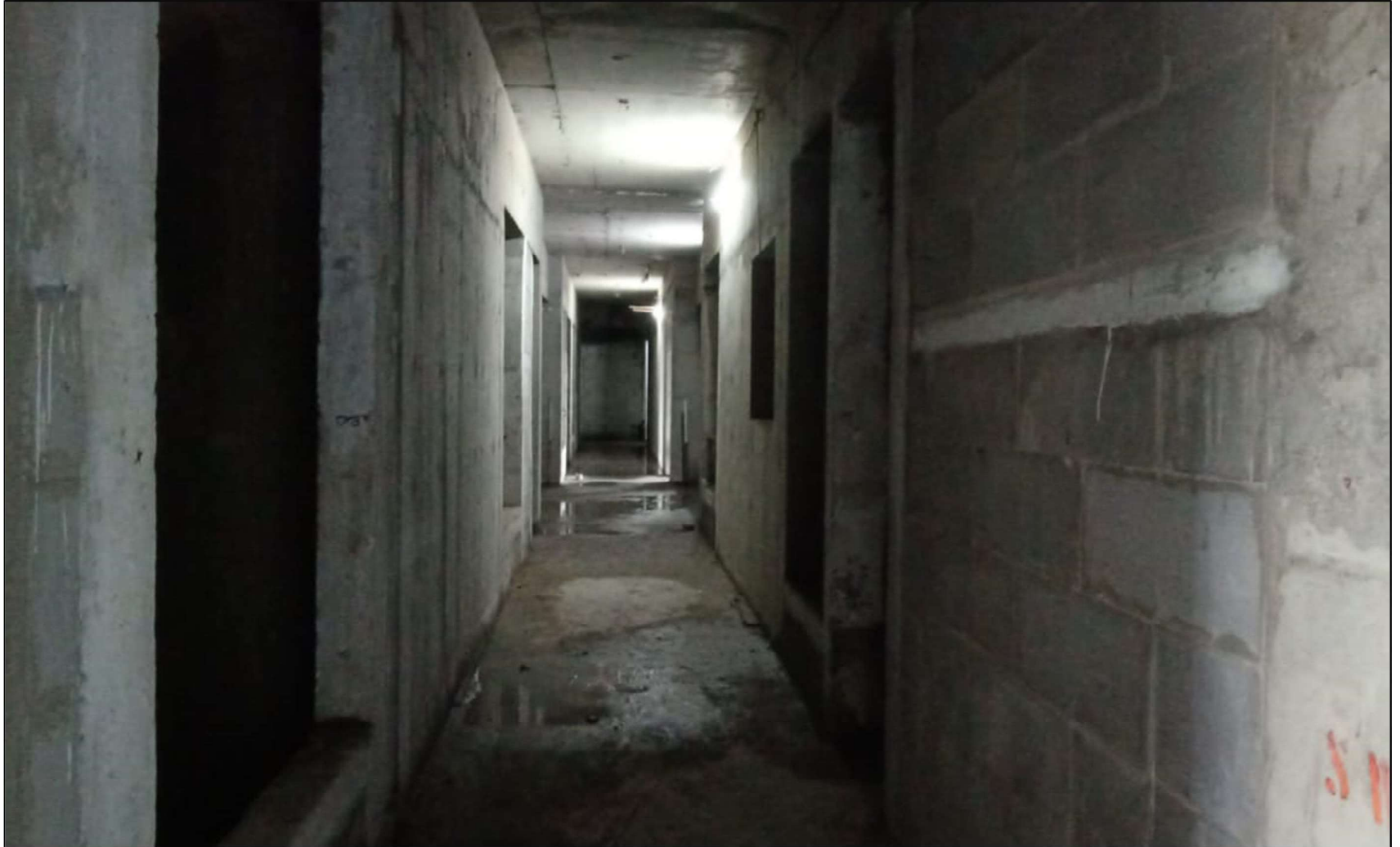
5 th Floor works under progress
