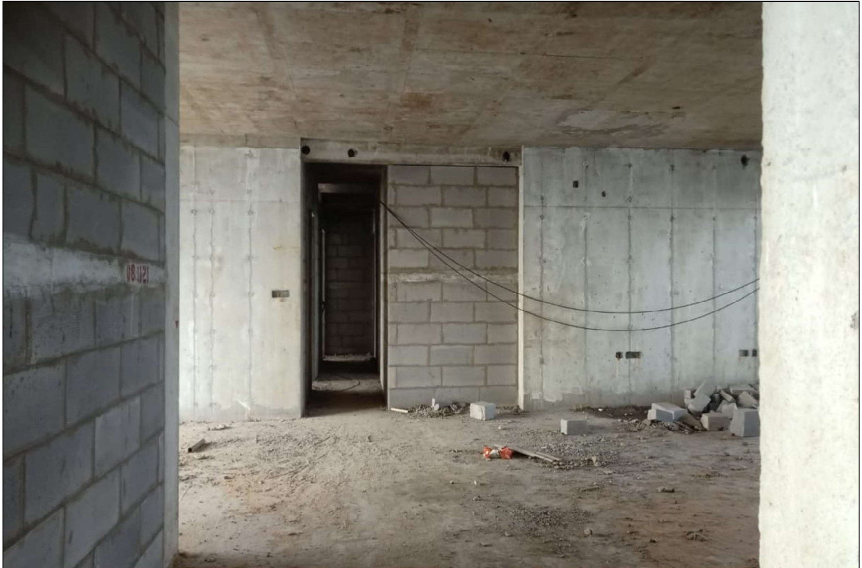
5 th Floor works under progress
