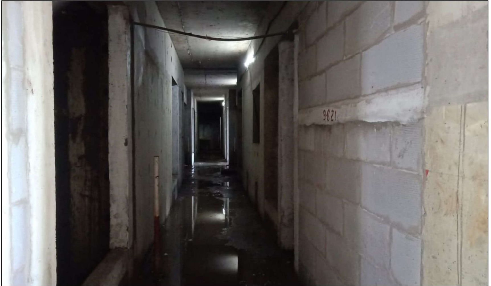
6 th Floor works under progress
