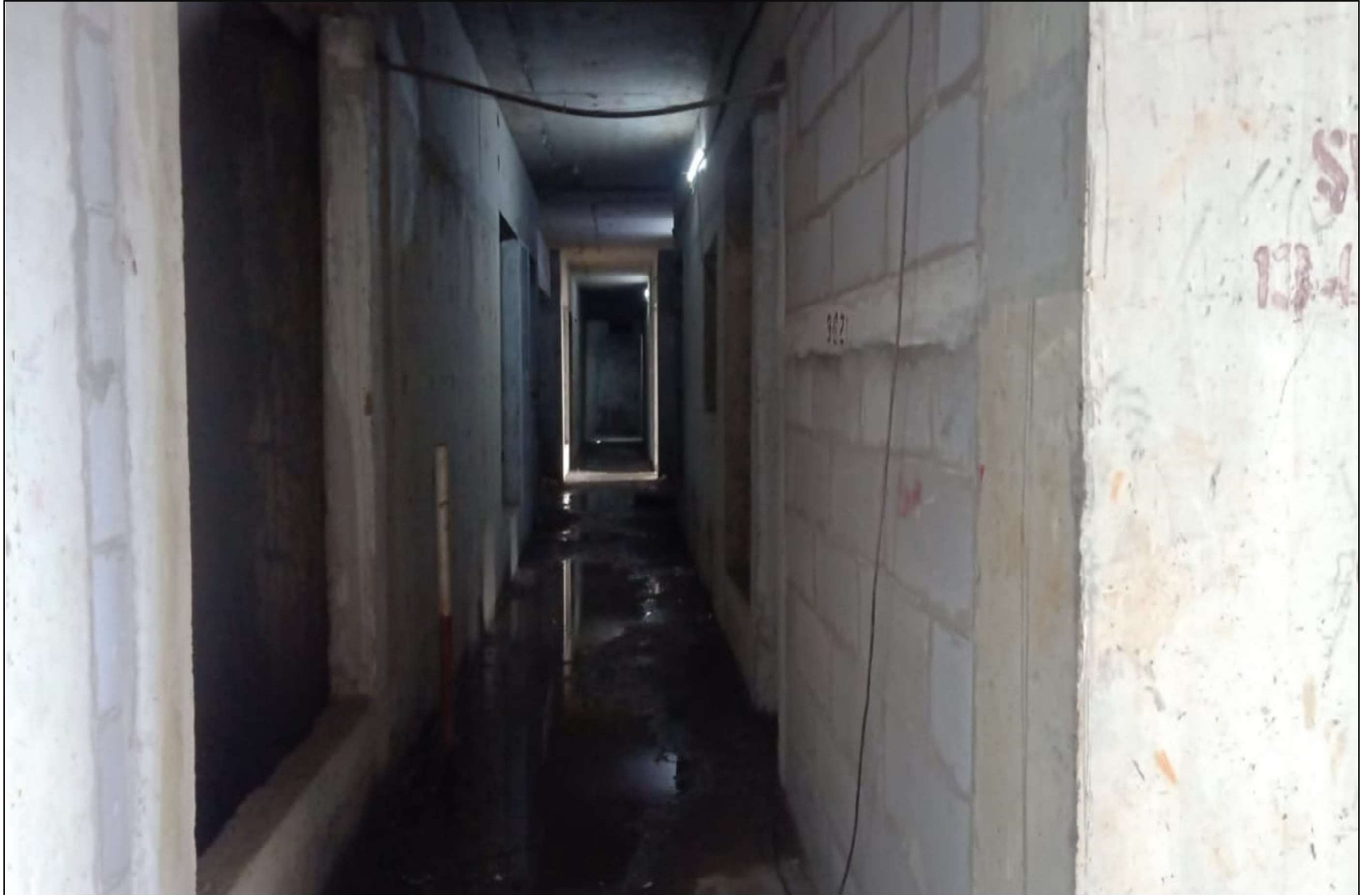
6 th Floor works under progress
