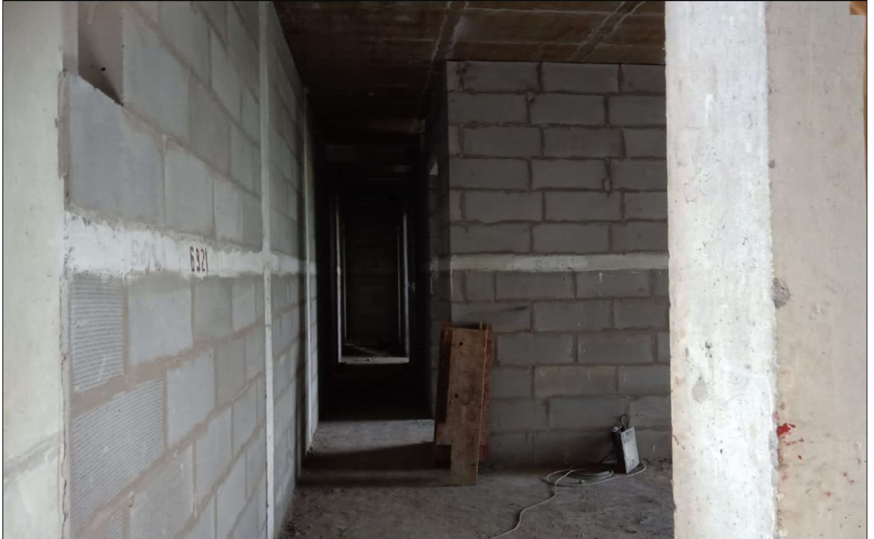
7 th Floor works under progress
