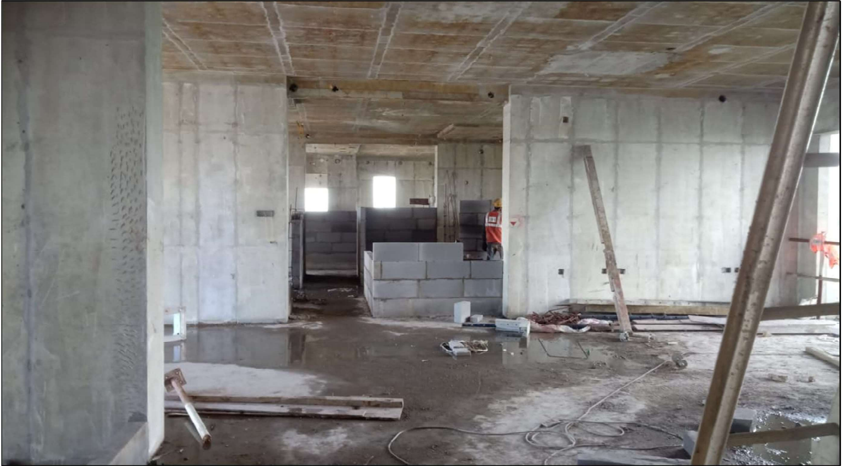
8 th Floor works under progress
