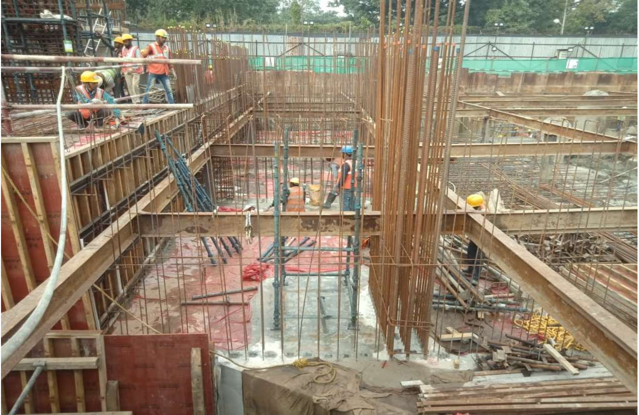
RAFT WORKS UNDER PROGRESS
