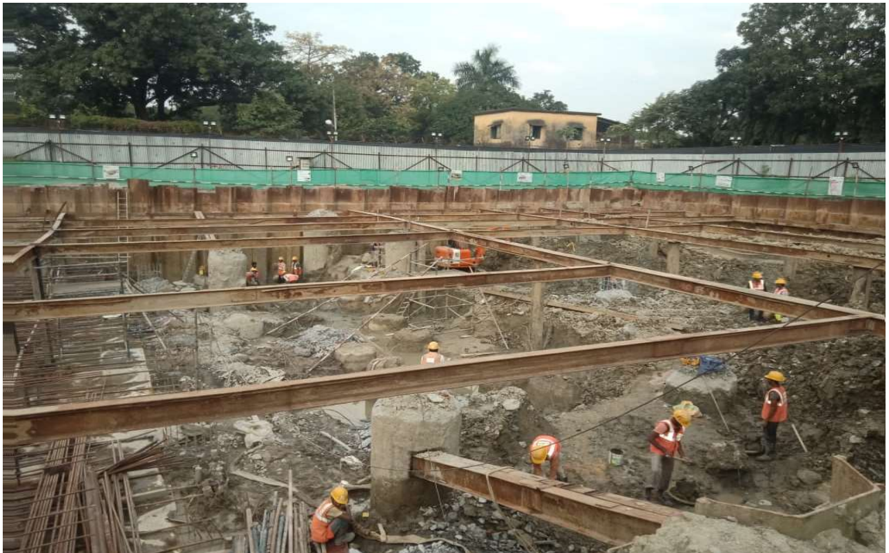
EXCAVATION WORKS UNDER PROGRESS
