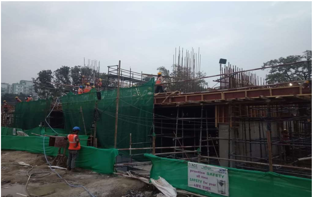
SLAB WORKS UNDER PROGRESS
