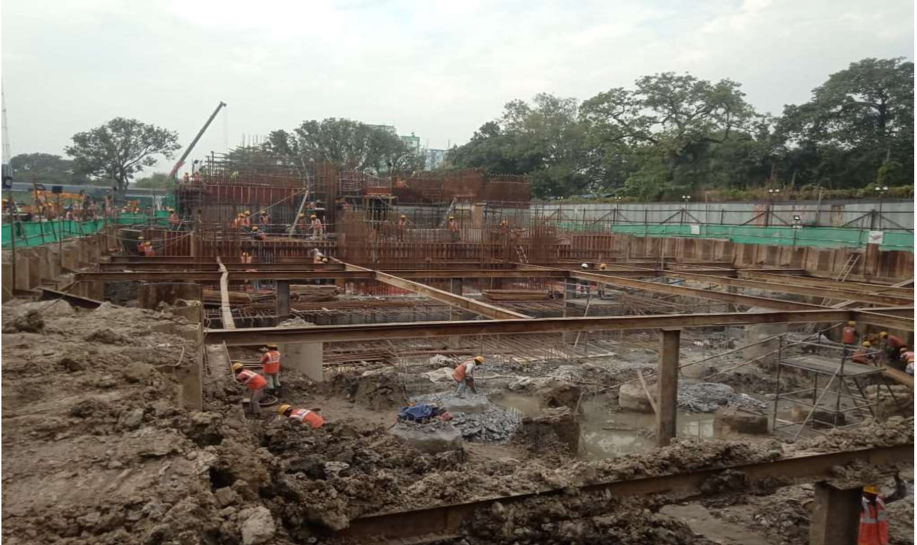
EXCAVATION WORKS UNDER PROGRESS
