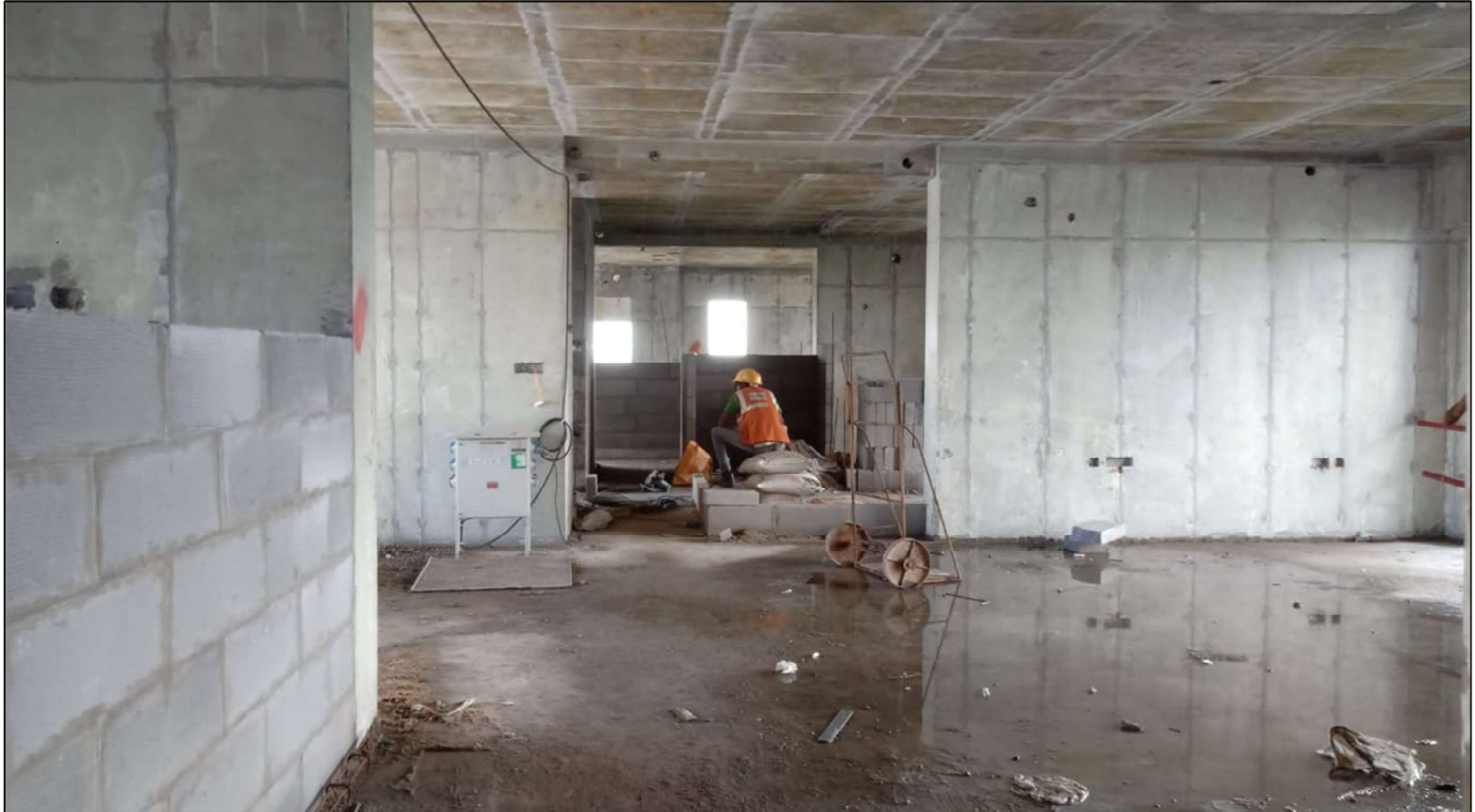
9 th Floor works under progress
