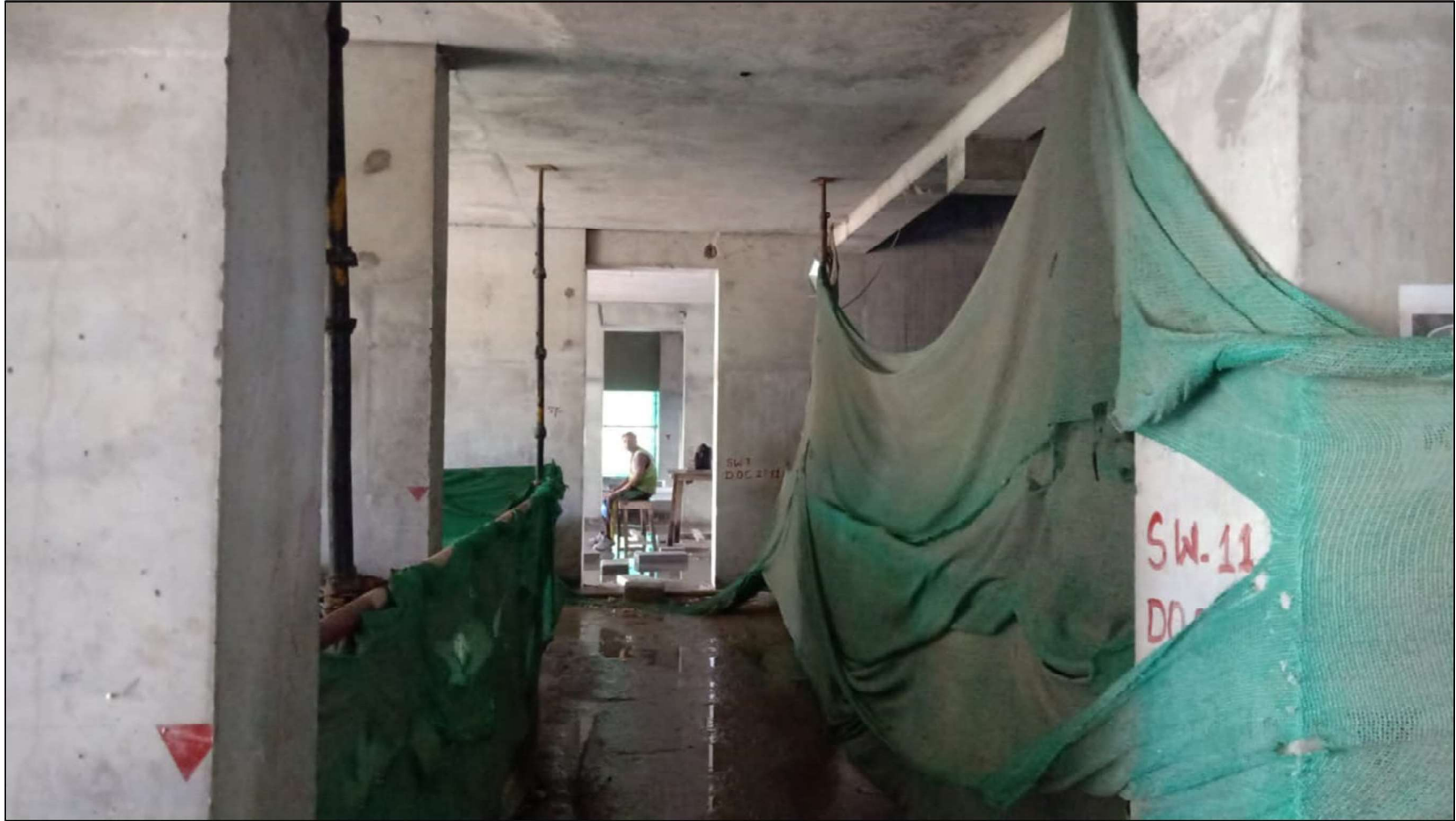
Ground Floor works under progress
