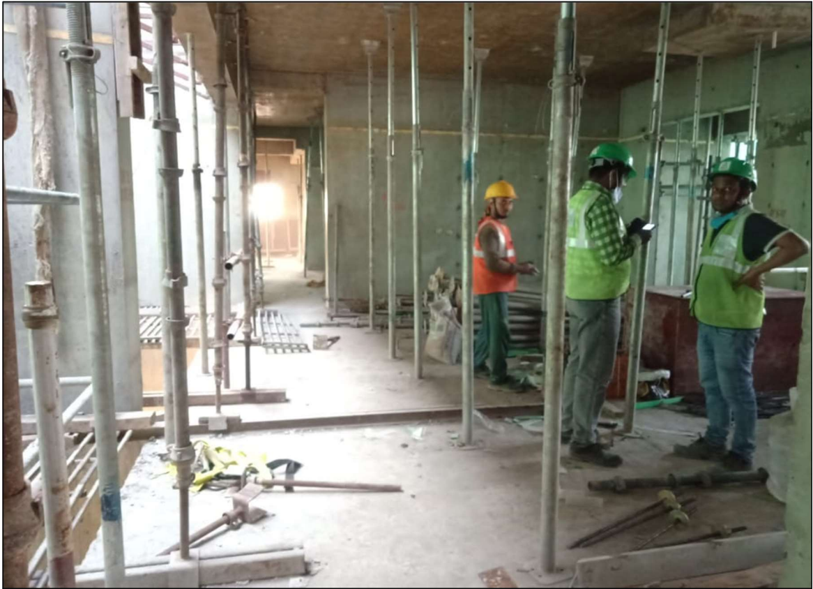
4 th Floor works under progress
