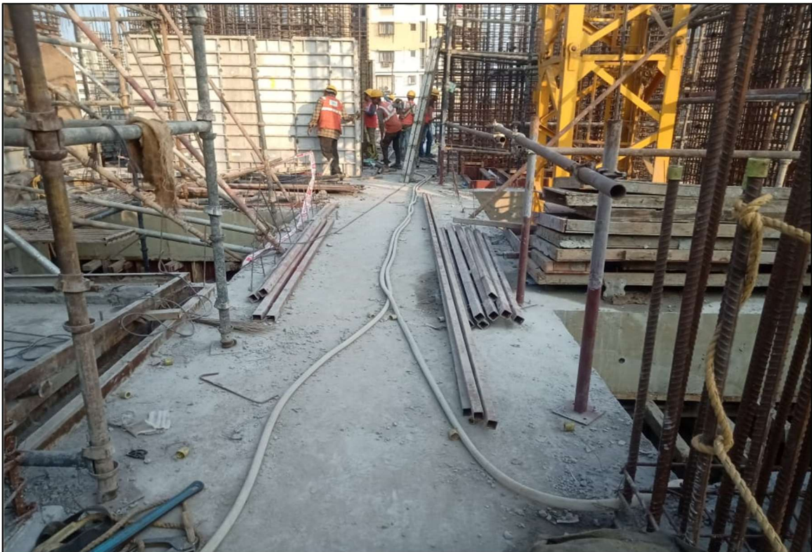
5 th Floor works under progress
