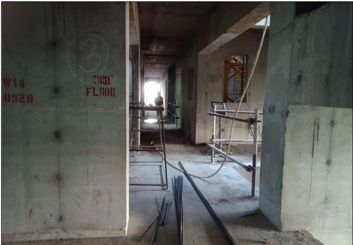
3 rd Floor works under progress
