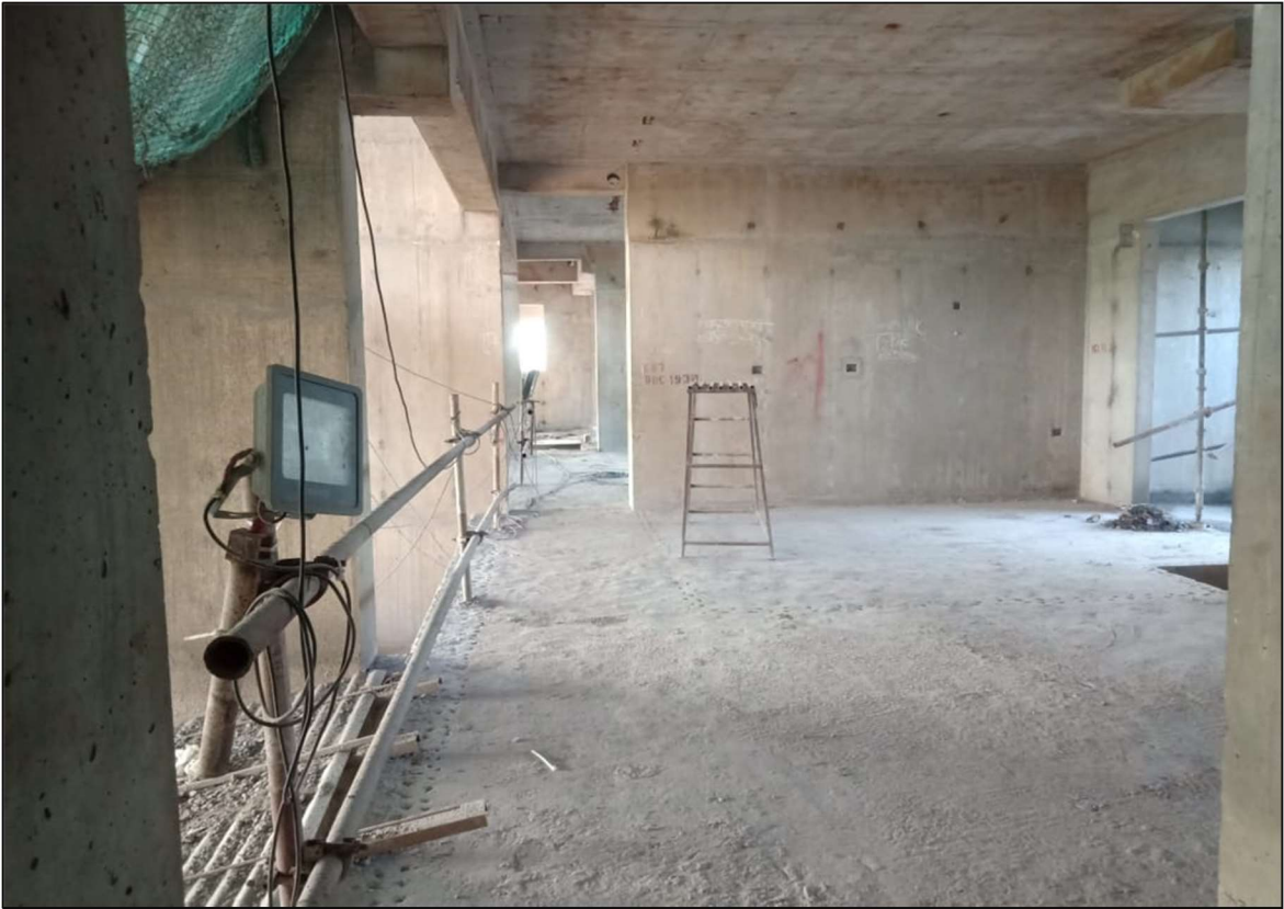
2 nd Floor works under progress
