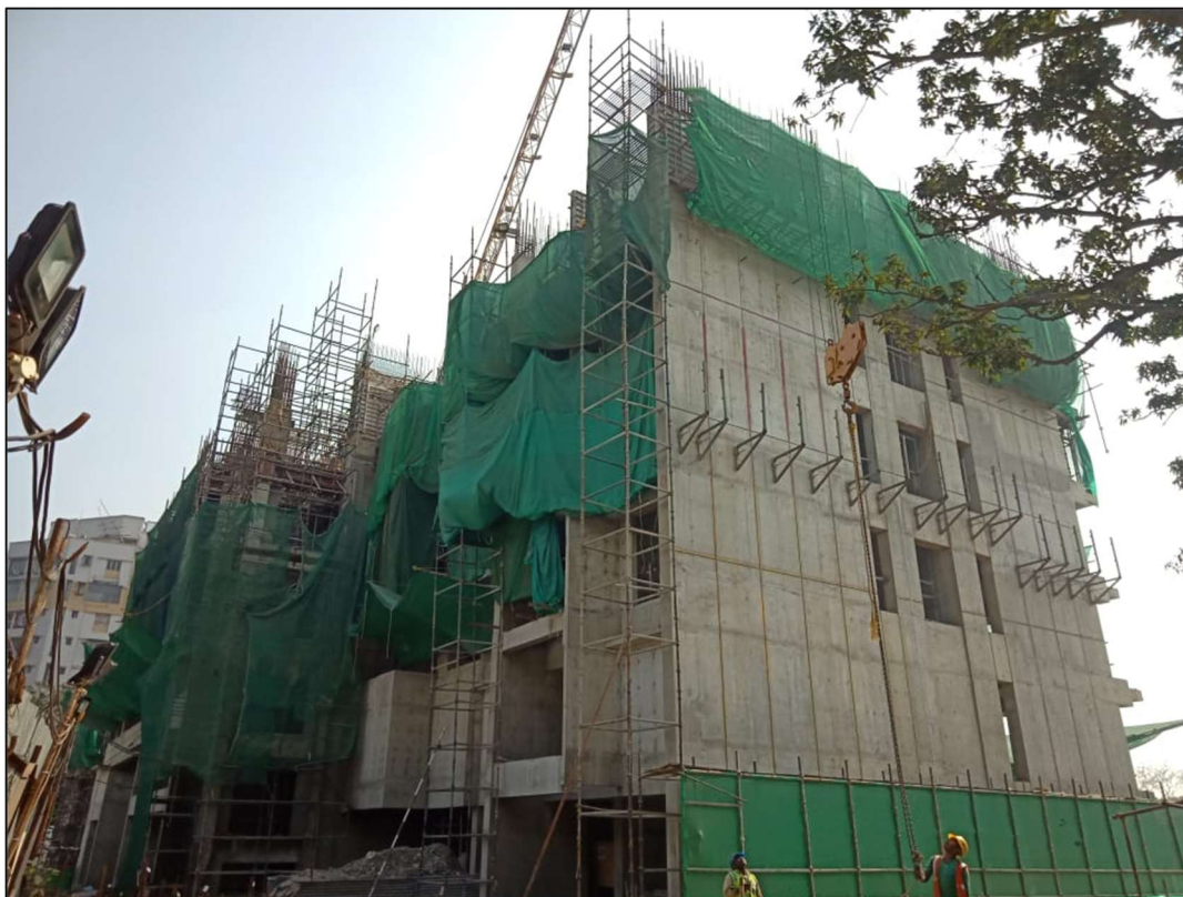
Tower area Shear Walls & Slab under progress
