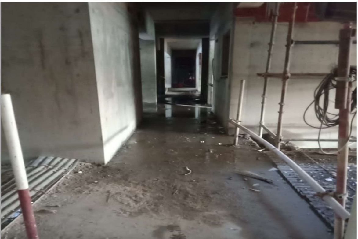
1 st Floor works under progress
