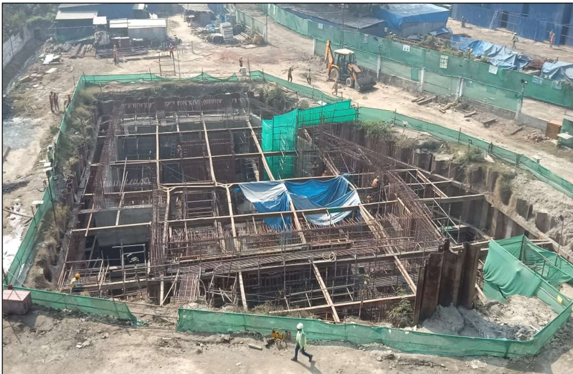
STP area works under progress
