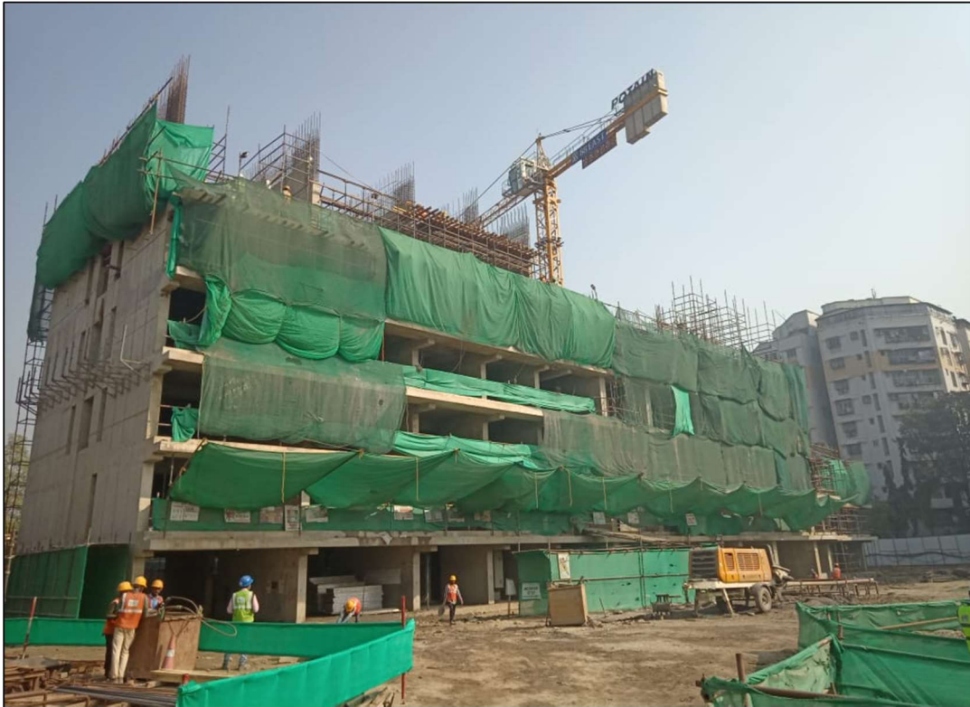
Tower area Shear Walls & Slab under progress
