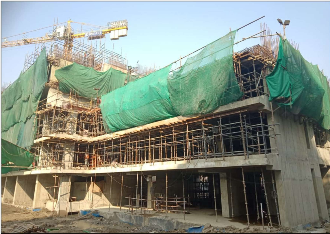
Tower area Shear Walls & Slab under progress
