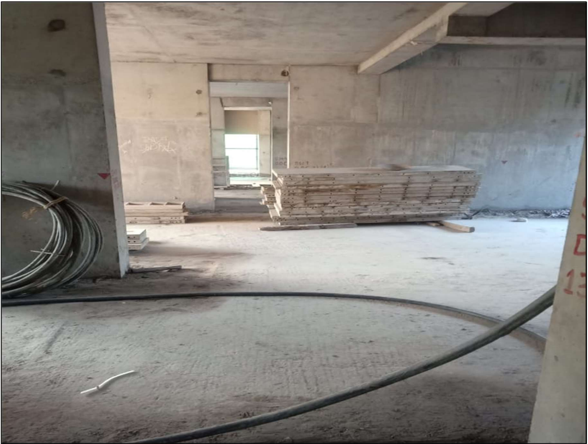
Ground Floor works under progress
