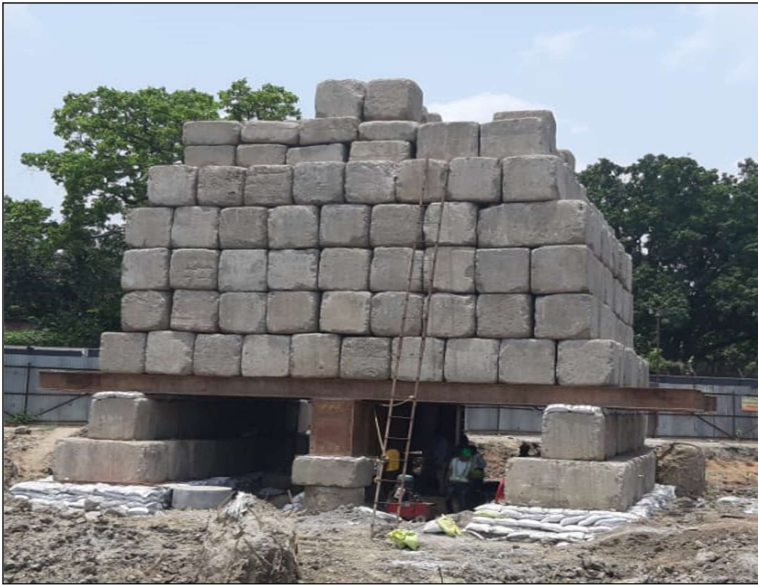
Pile Vertical Load Test Arrangement
