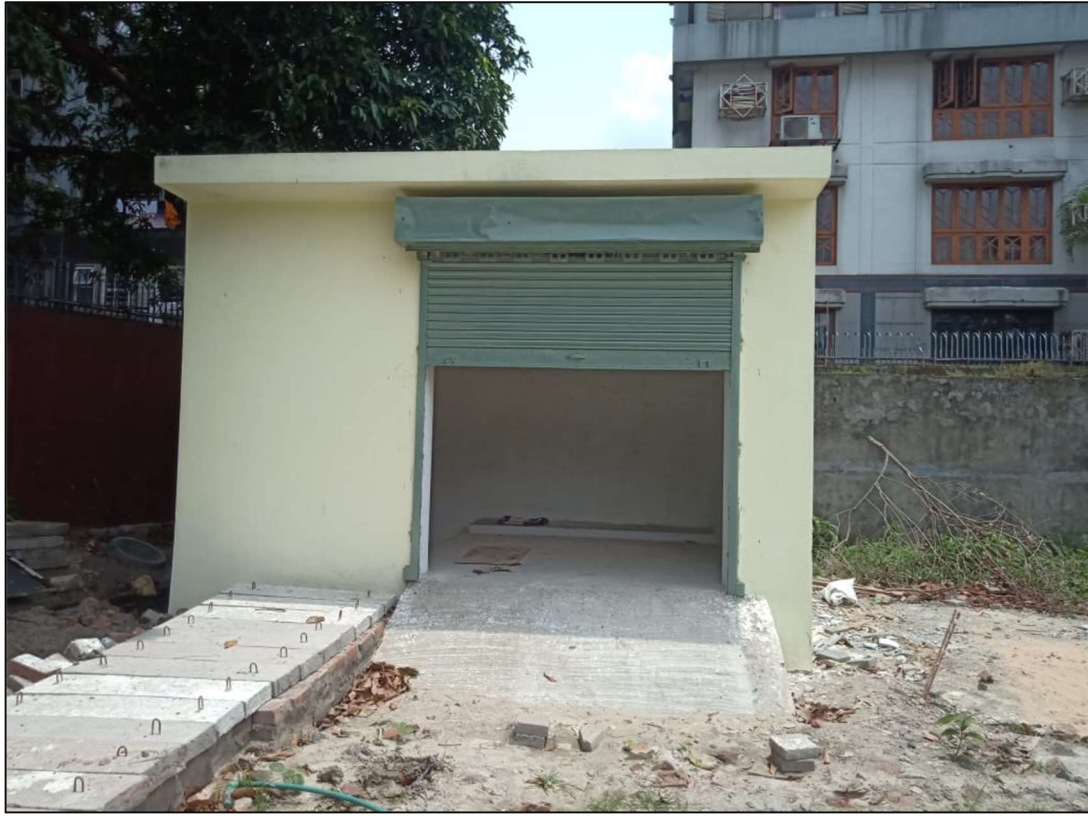
Temporary Substation Room
