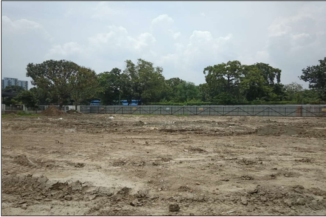
Piling Works Completed
