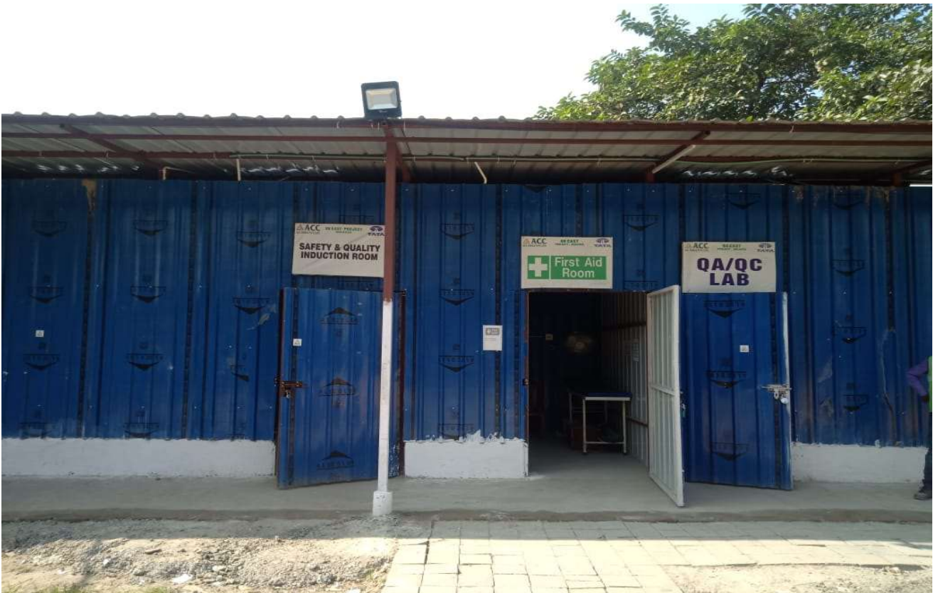
SITE SAFETY & QUALITY INDUCTION ROOM & QA-QC LABORATORY
