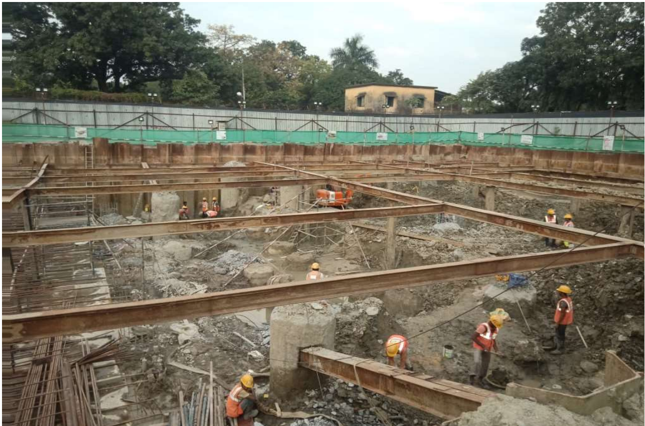
EXCAVATION WORKS UNDER PROGRESS
