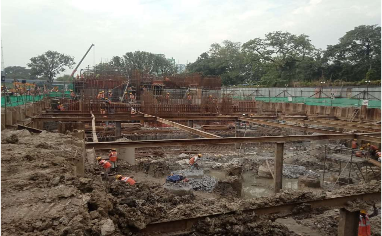
EXCAVATION WORKS UNDER PROGRESS
