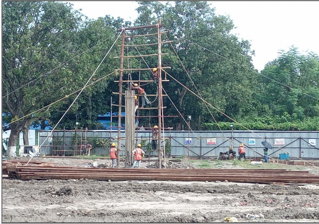
Shoring works (with ISMB 300 & 6 mm plate) completed
