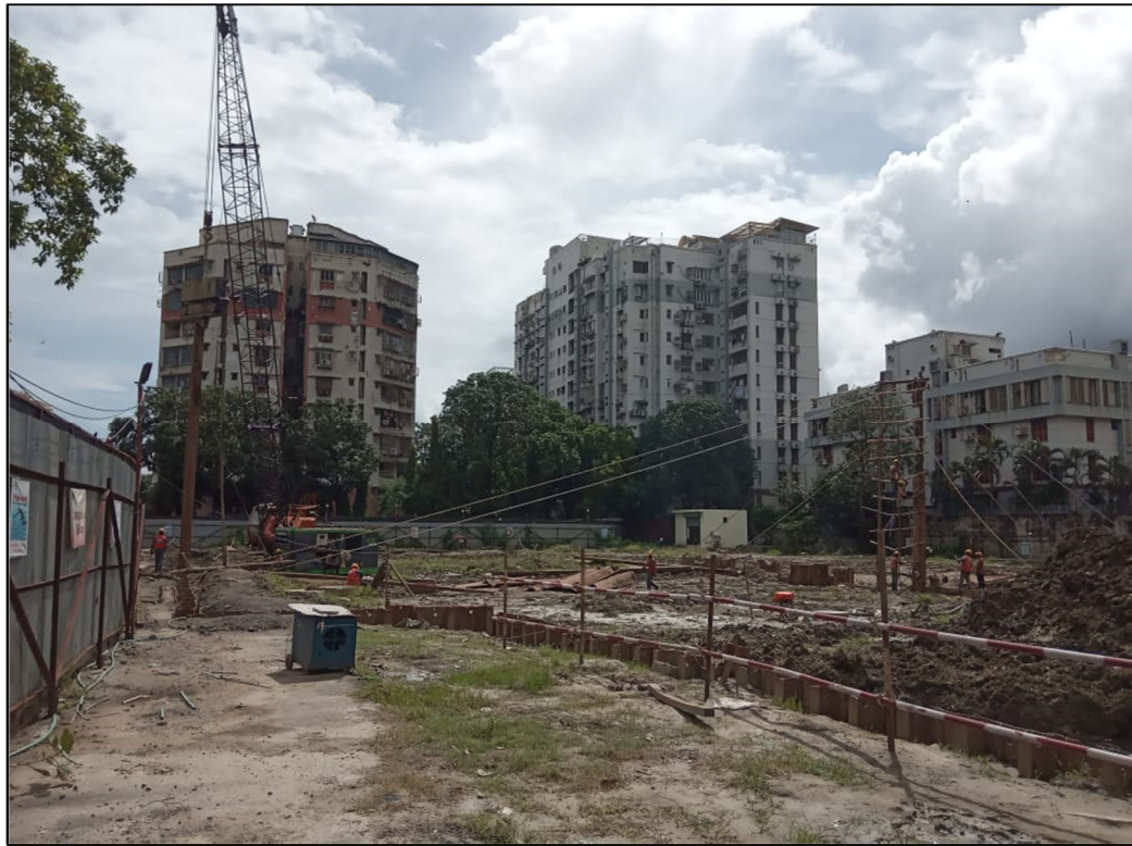
Shoring works (with Z-section) under progress
