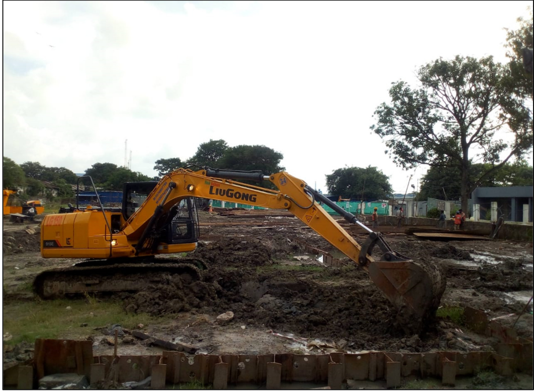
Excavation works under progress
