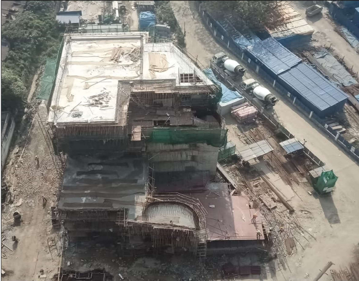
Podium above STP area works under progress
