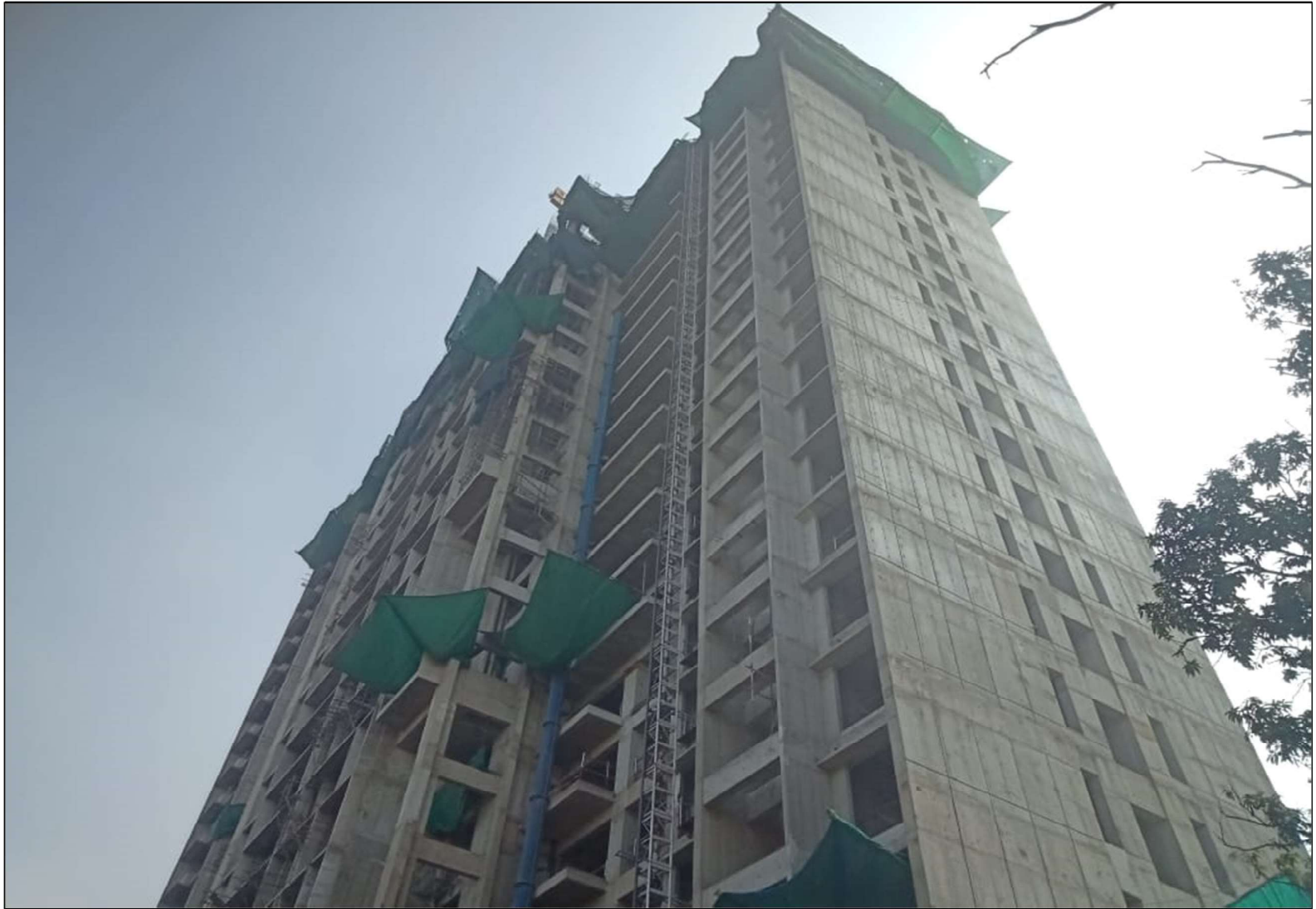
Tower area Shear Walls & Slab under progress
