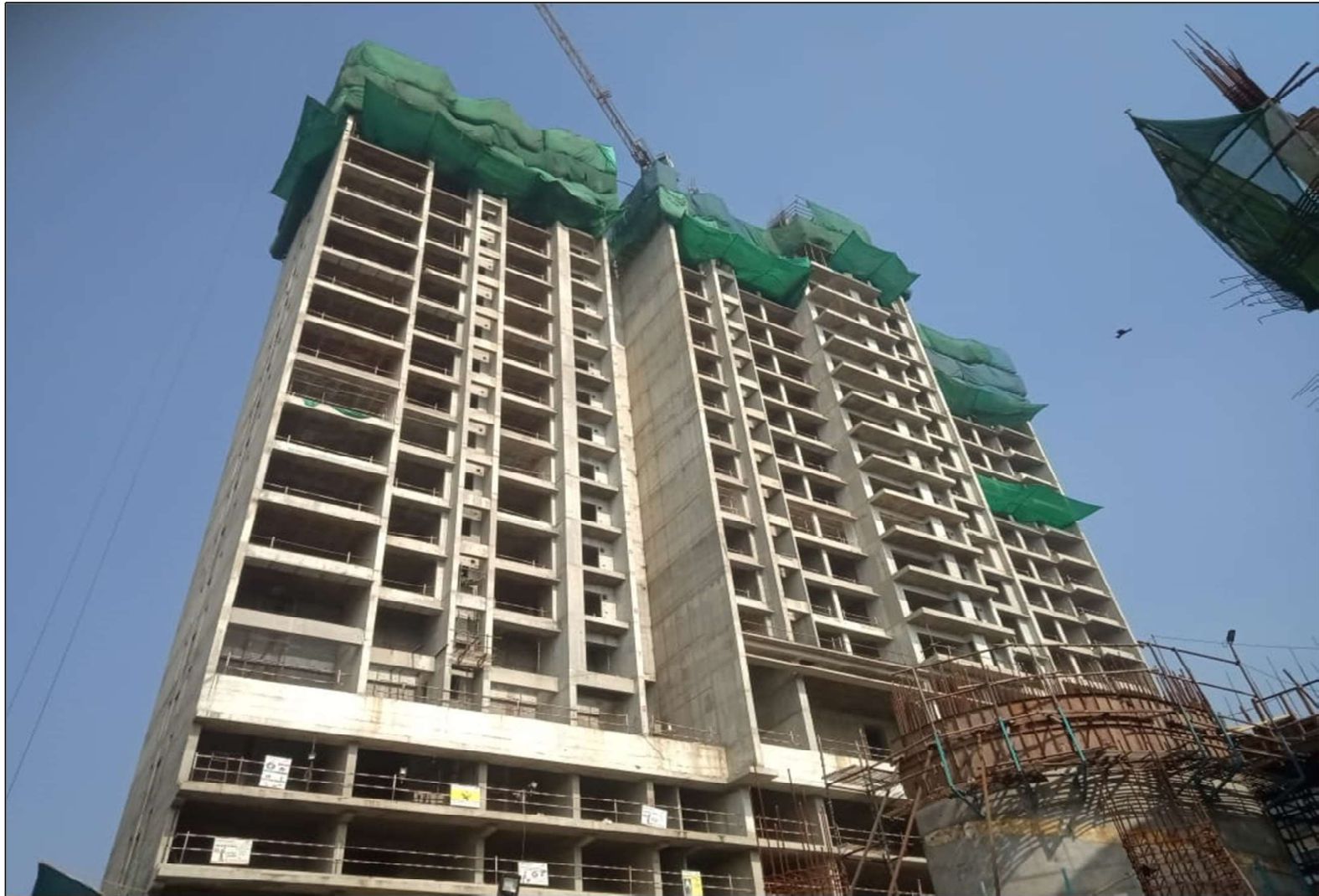
Tower area Shear Walls & Slab under progress
