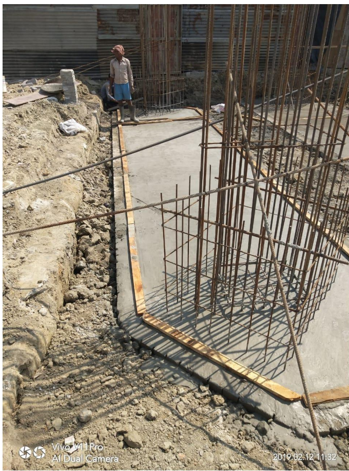
Picture 1 - Pile Cap
