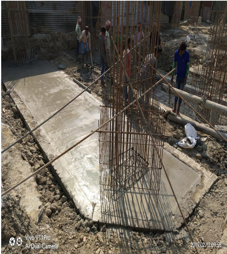
Picture 2 – Pile Cap
