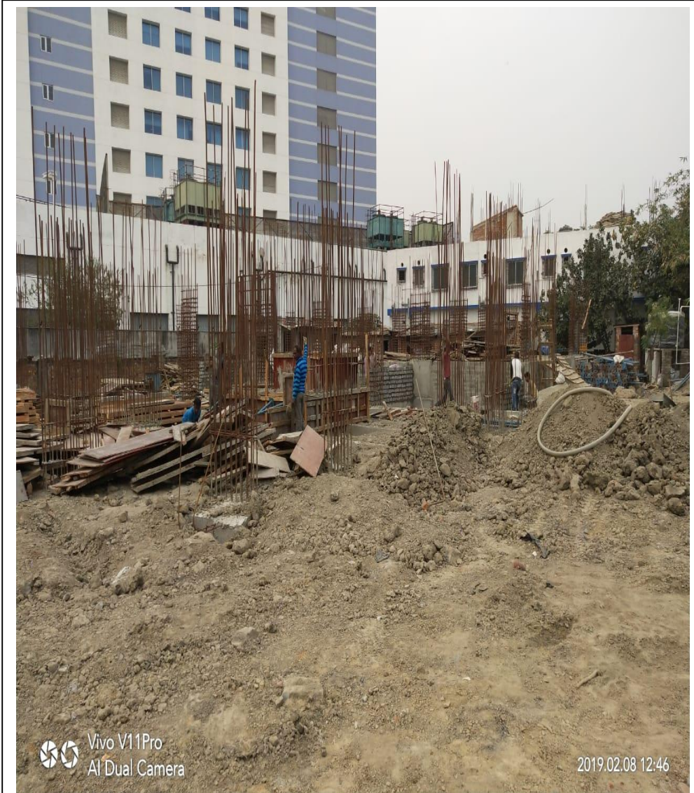
Picture 3 – Foundation Work
