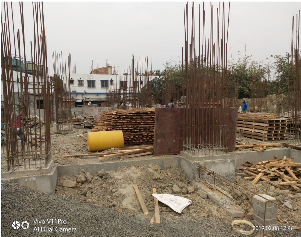
Picture 4 – Foundation Work
