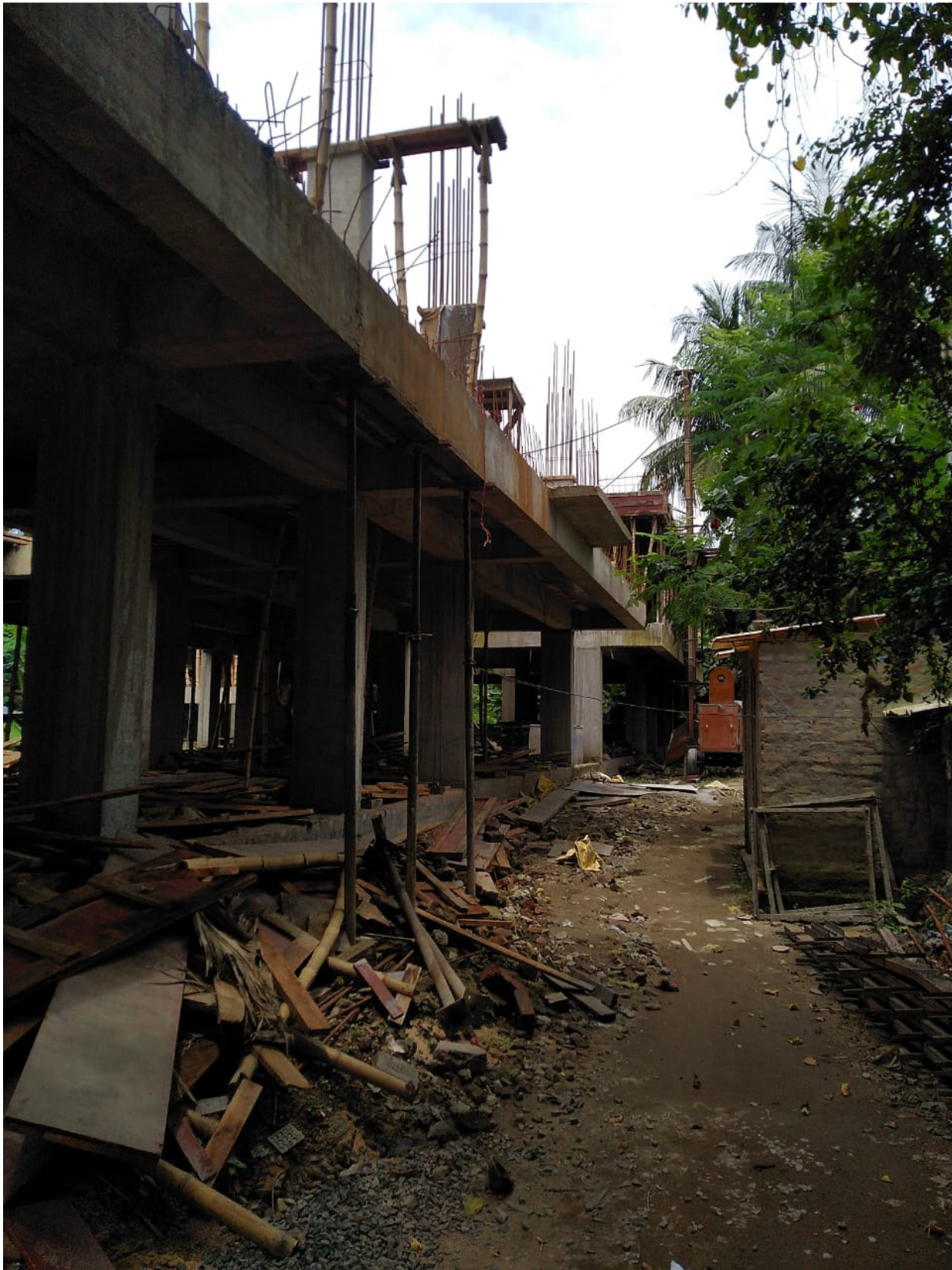
GLOBAL RESIDENCY_1 st FLOOR ROOF CASTING WORK UNDER PROGRESS
