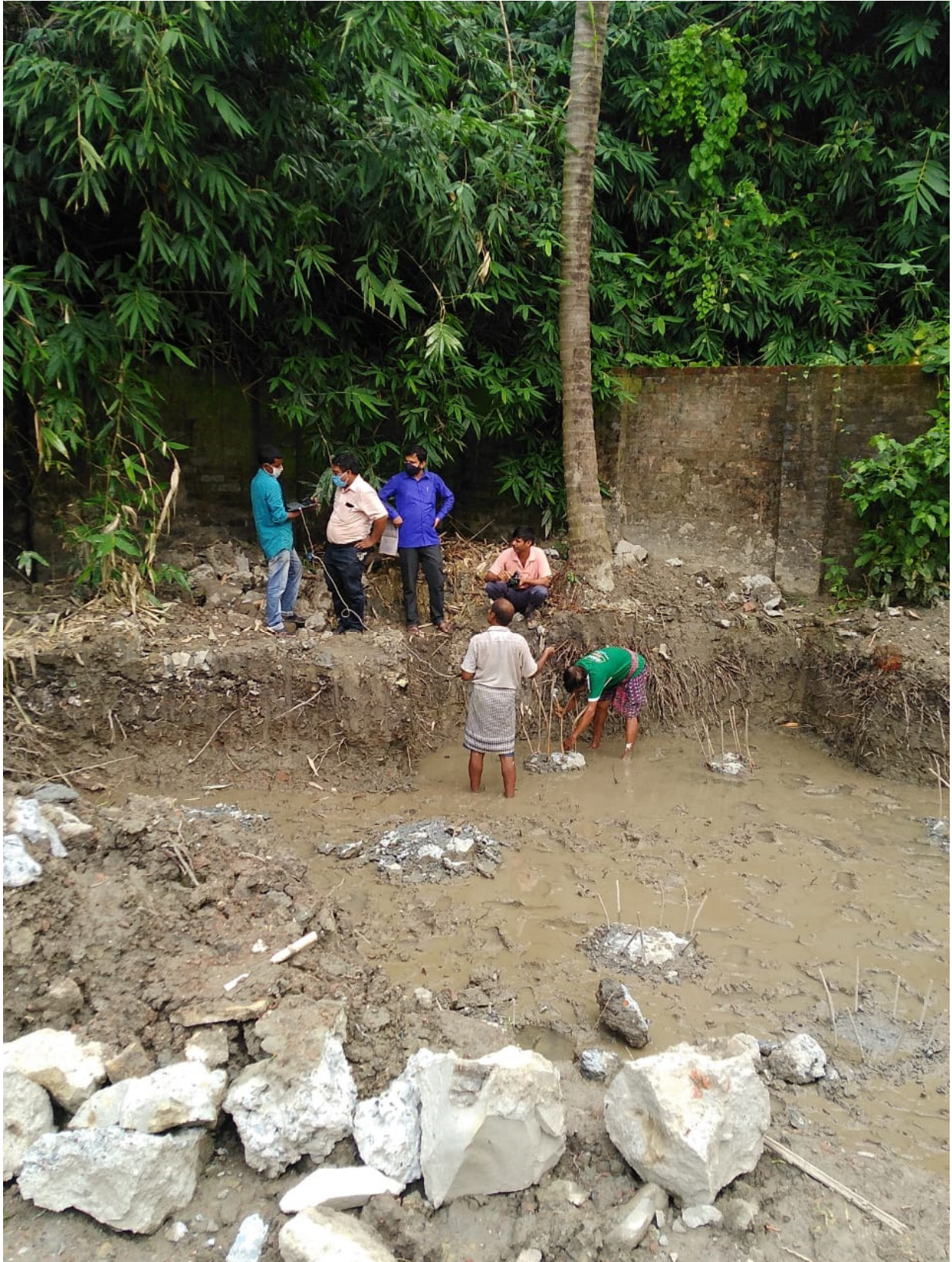
GLOBAL RESIDENCY_PILE LOAD TESTING & FOUNDATION WORK IN PROGRESS
