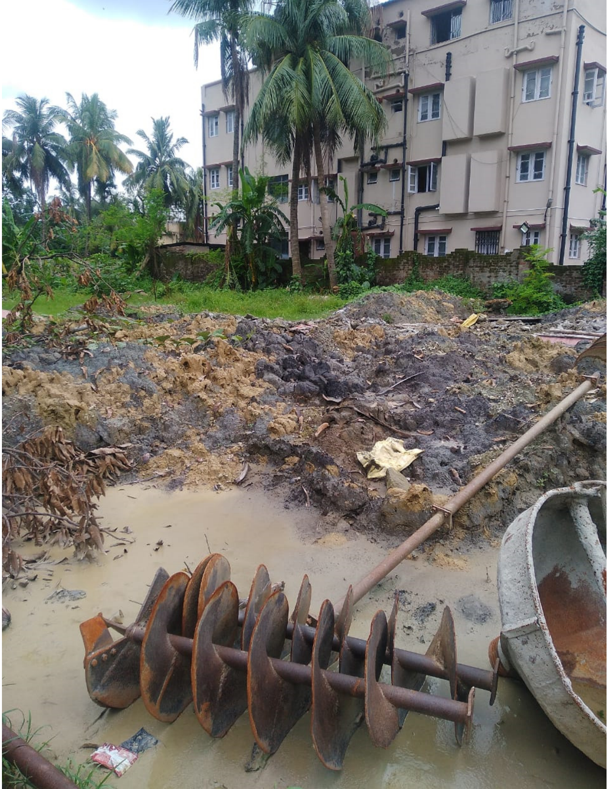
PILING WORK IN PROGRESS
