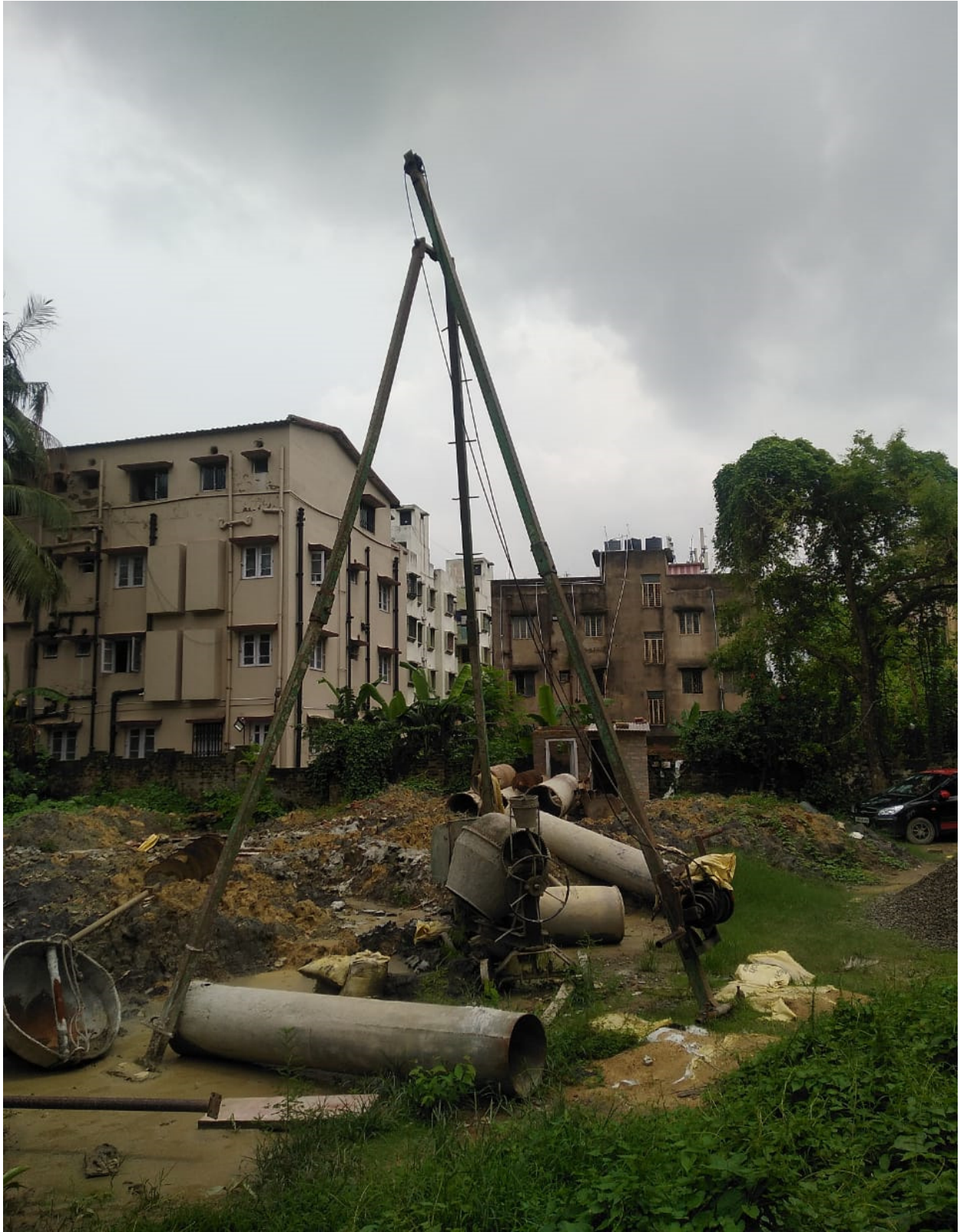
PILING WORK IN PROGRESS
