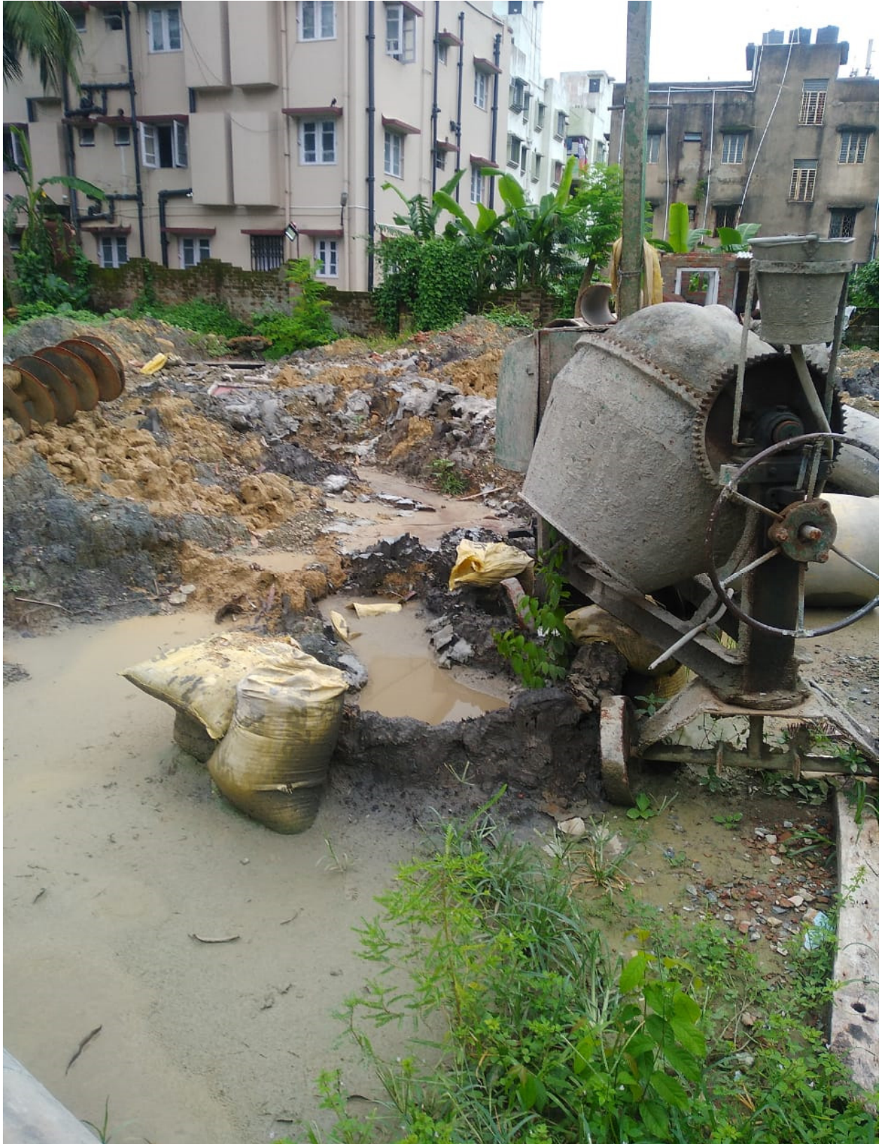
PILING WORK IN PROGRESS
