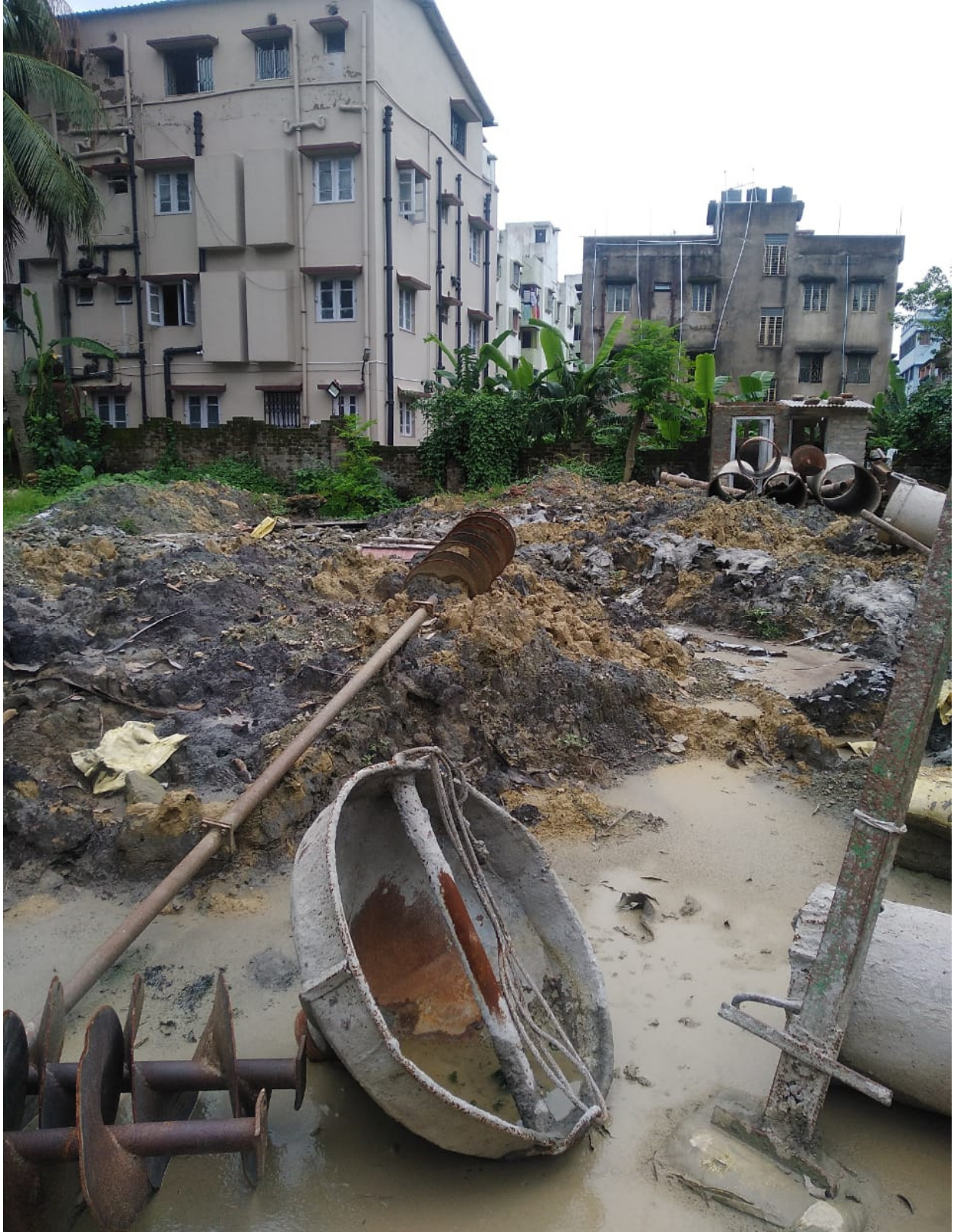
PILING WORK IN PROGRESS
