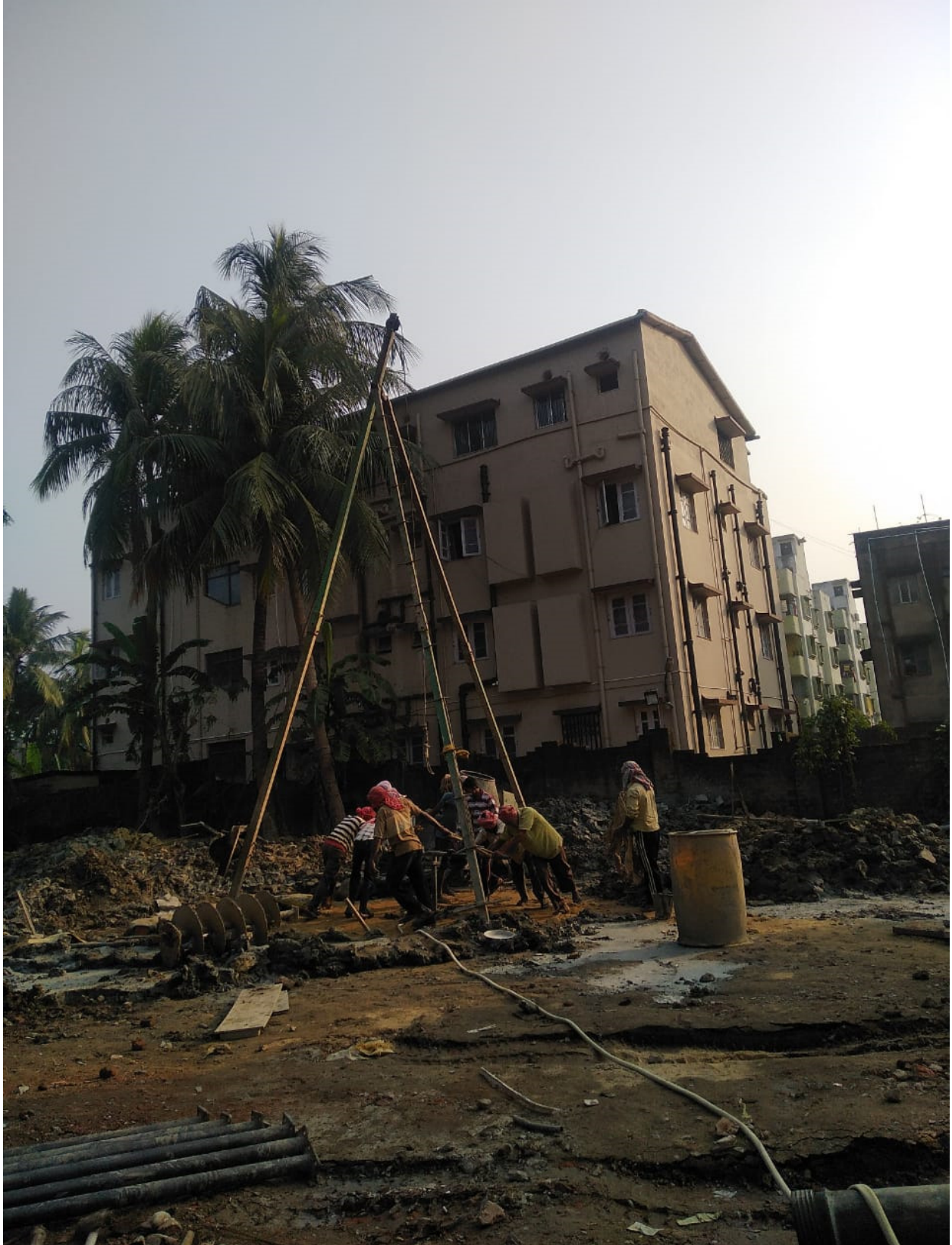
PILING WORK IN PROGRESS
