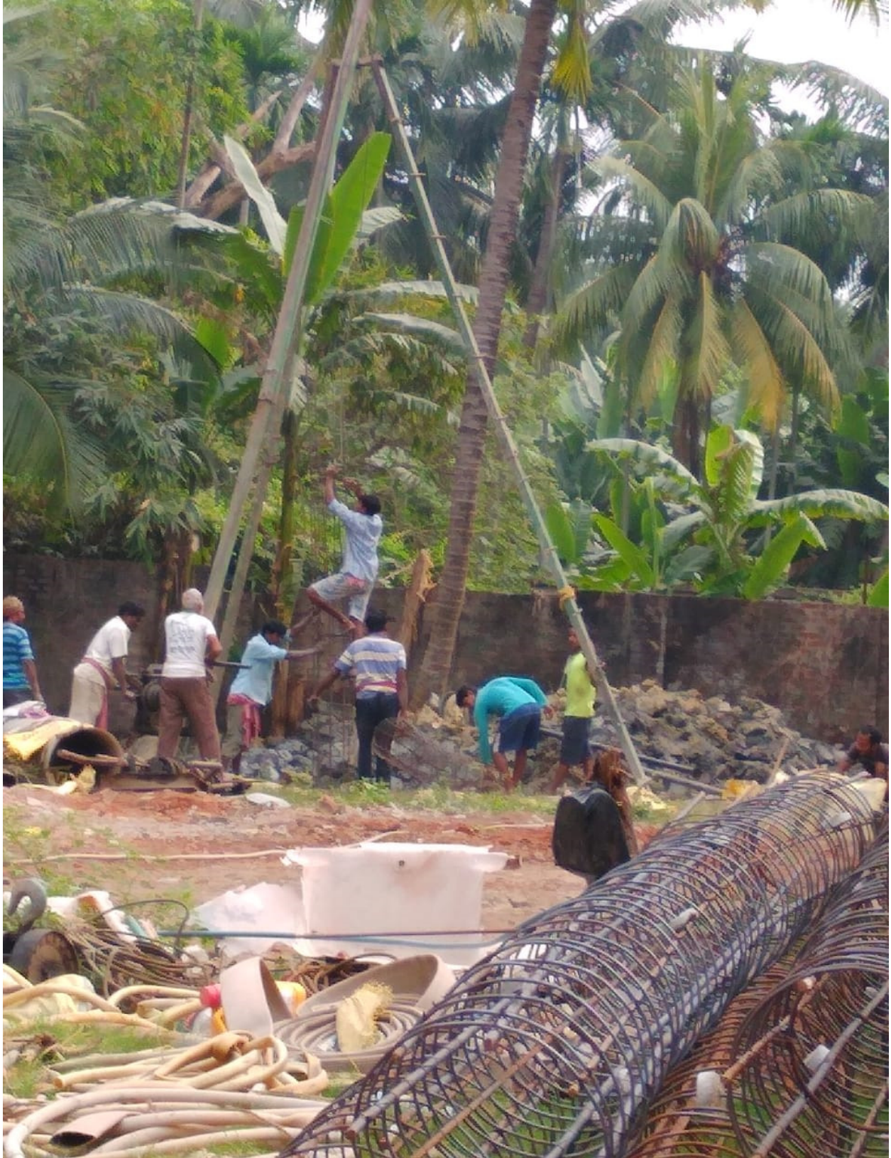
PILING WORK IN PROGRESS
