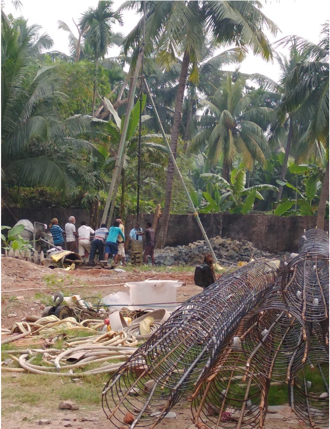
PILING WORK IN PROGRESS
