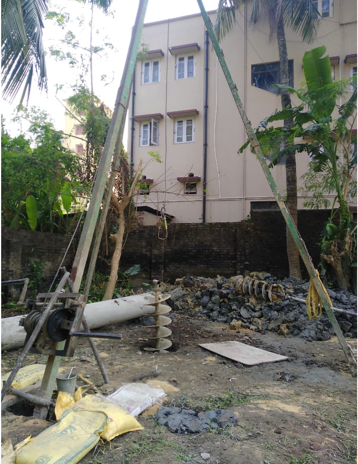
PILING WORK IN PROGRESS
