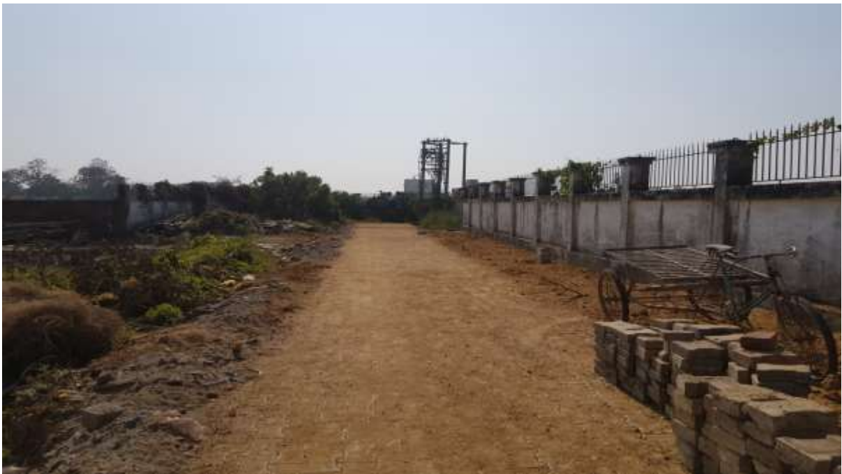
WBSEDCL Power Transformer with approach Road.(315 KVA)
